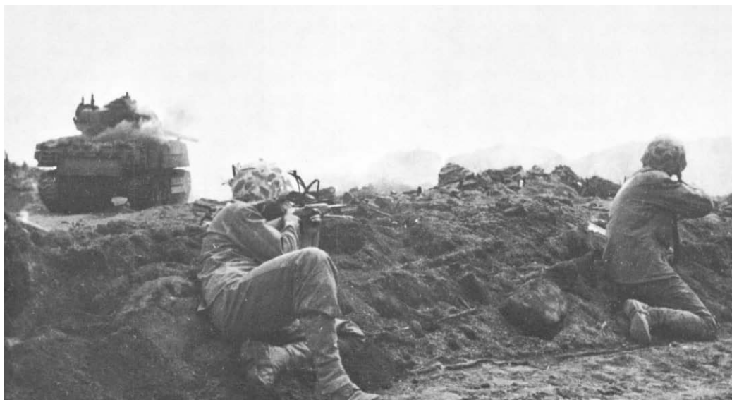
ENEMY POSITIONS near Nishi Village under fire. Note burning M-4 tank at left. (USMC 142316)
