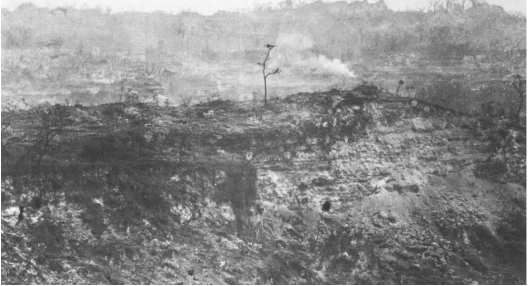
WANA RIDGE , rugged barrier in the path of the 1st Division, is shown looking southeast toward Shuri. (USMC 148651)
