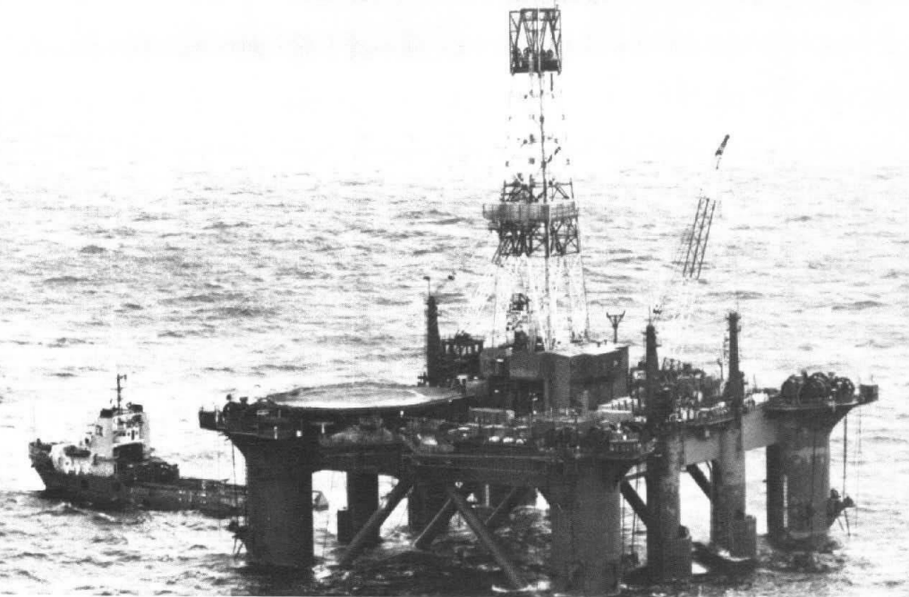
Finnish-built oil-drilling rig Dyvi Delta in the North Sea Courtesy Embassy of Finland, Washington
