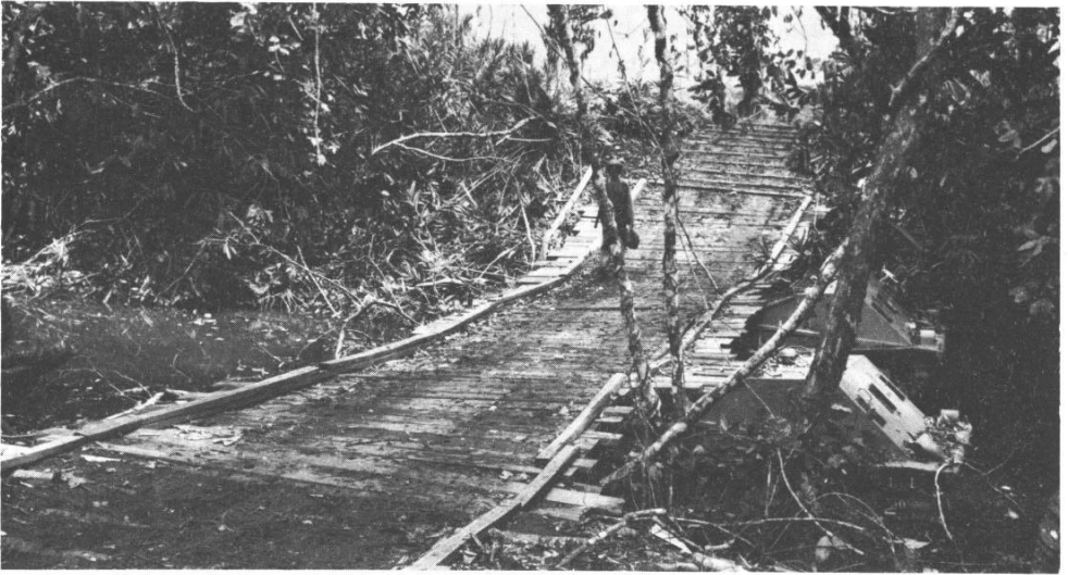
MARINE ENGINEERS erected this bridge across the Tenaru River to speed the flow of troops and supplies from the beaches to the perimeter. (USMC 50468-A)
