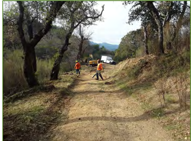
Photo 15: Roadside Mowing at Upper Shaver Grade.
