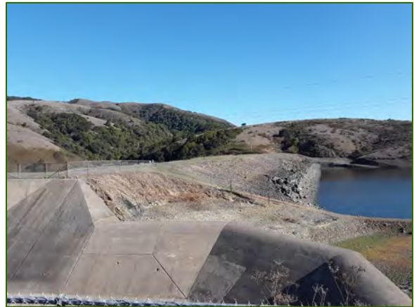
Photo 17: Dam maintenance at Soulajule Dam.
