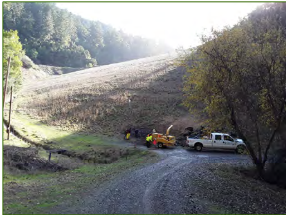
Photo 16: Dam Maintenance at Peters Dam.
