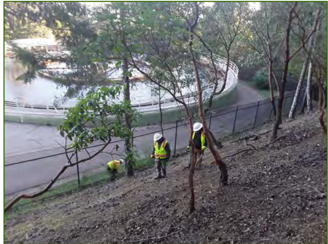
Photo 11: Routine Fuelbreak Maintenance at Bon Tempe Treatment Plant.
