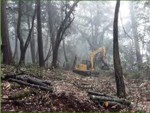
Photo 22: During completion of forest restoration work near Mt. Theater.
