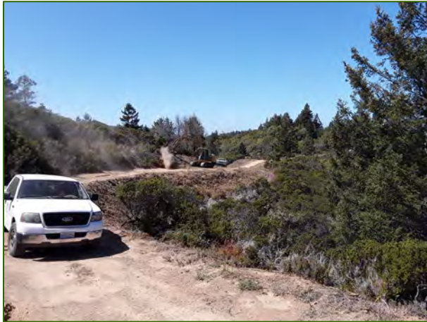
Photo 14: Roadside Mowing at Pine Mt Fire Rd.
