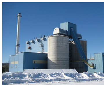
Springfield power plant (New Hampshire, USA)
