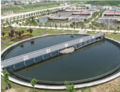
Wastewater treatment site in Changsha (Hunan Province, China)
