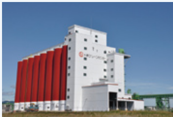
Large grain silo at Tokachi Grain Terminal Co., Ltd.
