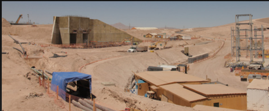
Processing site for the Esperanza copper mine when under construction
