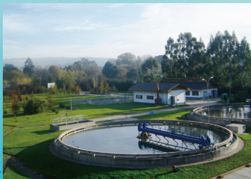
Wastewater treatment plant in Valdivia, Chile
