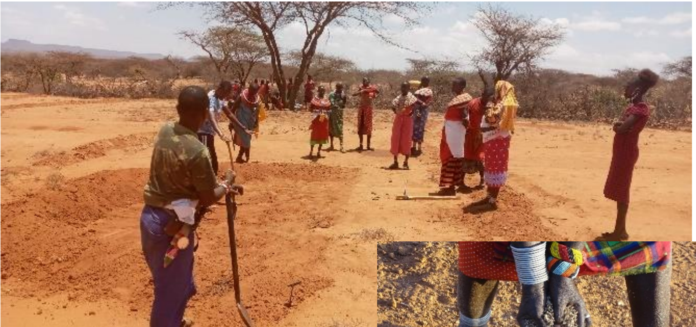
Pics. 08: Community members from Remot village, Westgate Conservancy, constructing semi-circular bunds © GZT
