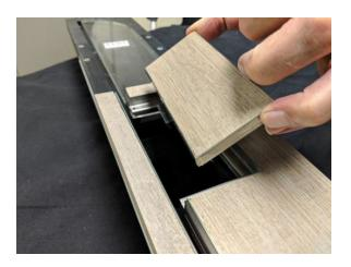
8. Re-Install the Access Cover by angling the cover down to the Drain Channel until the ball detents catch the Access Cover Frame. Push the cover down until flush.
