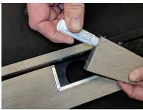
7. Before re-installing the Access Cover apply wax or petroleum jelly around perimeter to aid in future removal.
