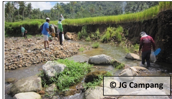
f. Collapsed of rice paddy (Tigbao Creek)
