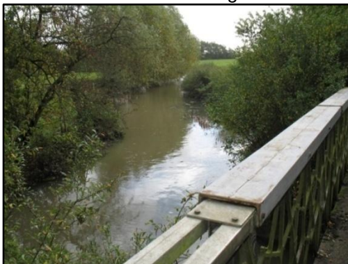
River Anker at Caldecote Bridge (looking North)
