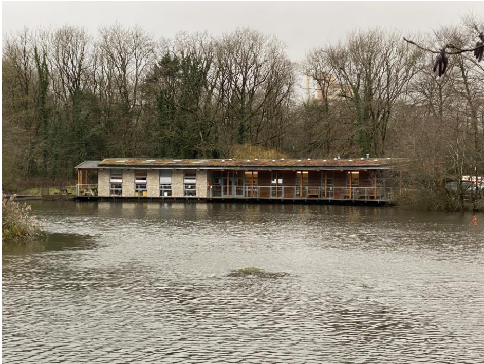
Figure 12 – The Earth Science Centre, Moon’s Hill Quarry. An educational and research facility sponsored by local aggregate producers. Opened in 2009 by the Princess Royal
