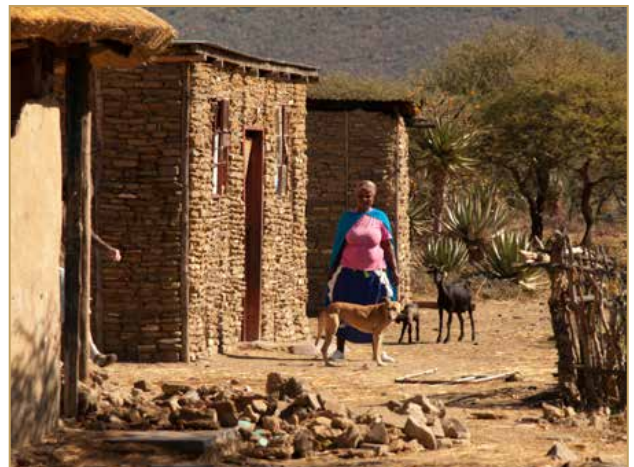
Imizi isiyakhiwa izinhlobo zezindlu ezixubile. Amafadi nolondo. Ezinye ngosimende ezinye ngodaka. Ezinye zifulelwe ngothayela ezinye utshani. Esekelwa ubaba wakhe, uMpembe, uSiphokuhle Mvelase wazakhela umuzi wakhe, futhi noma enawo "amafadi" wothayela, indlu yakhe yokuhlala yakhiwe ngodaka yase ifulelwa ngotshani.
