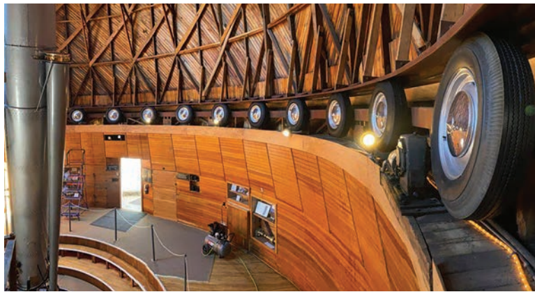
Vintage-looking Firestone tires were installed as part of renovations at the Lowell Observatory in Flagstaff, Ariz.
