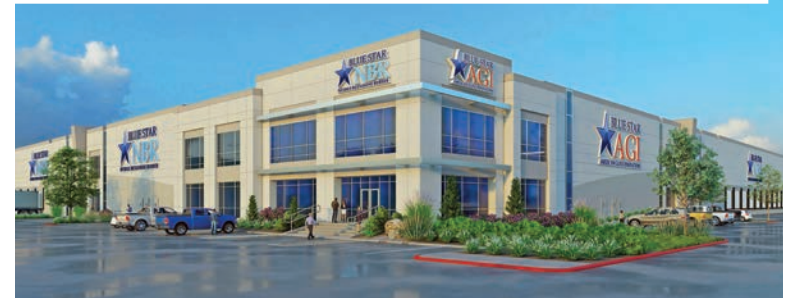
Blue Star NBR broke ground last month on a $714 million multi-facility operation that includes NBR and nitrile glove production facilities in Wytheville, Va.
