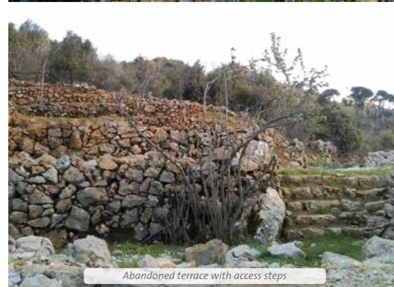
Degraded dry stone walls
