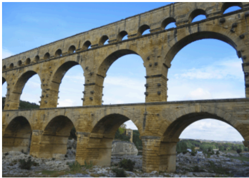
1. Aqueducts Modern example:
