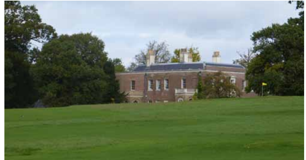
View of Morden Park House Road behind the undulating topography of the pitch and putt course
