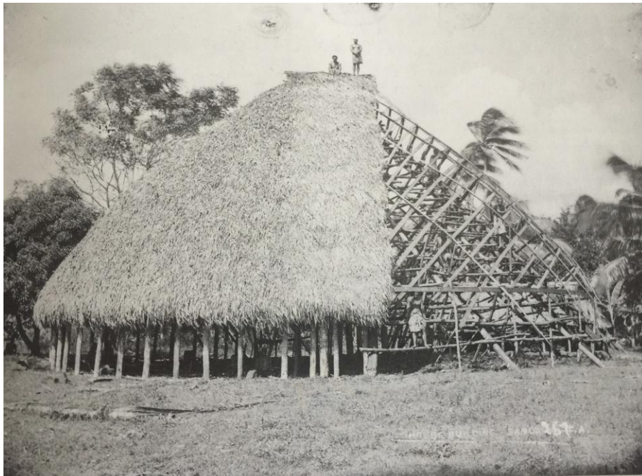
Figure 1: Samoan Faletele Under Construction circa 1900
