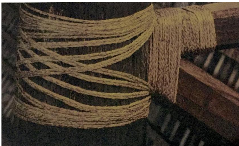
Figure 2: Rafter Lashing Sinalei Reef Resort photograph by Craig Potton
