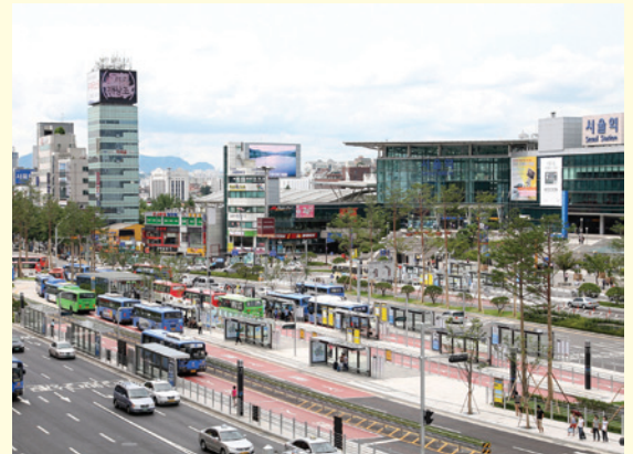
After [Seoul Station Transfer Center]
