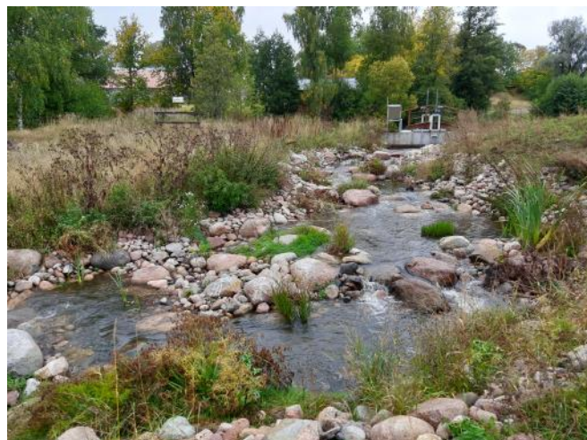
The Billnäs technical fishway in the construction phase (left) and the finished Koski semi-natural bypass (right).
