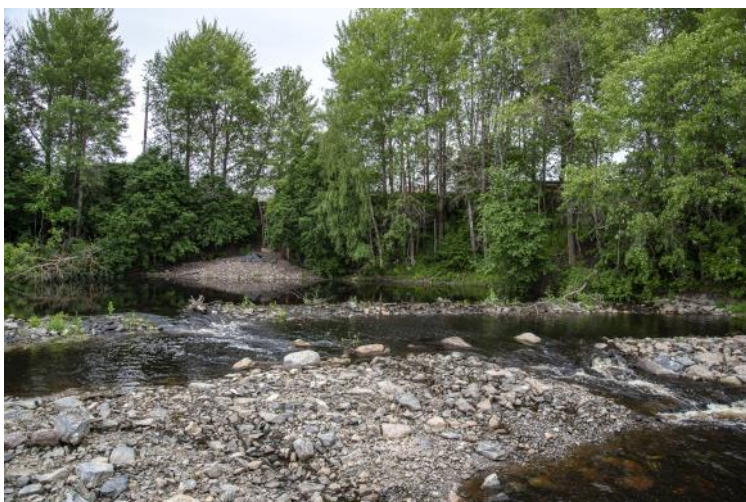
Constructed check dams above the former dam in Villamo, Isojoki.
