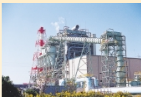
Nagoya Power Station of Nakayama Nagoya Kyodo Hatsuden Co., Ltd.
