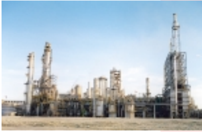
Ammonia Plant (Indonesia)
