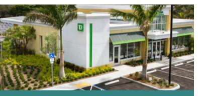
In 2011 TD Bank built a Zero Net Energy retail bank branch in Fort Lauderdale. The 3,970 square-foot building include several energy efficiency features such as a high-performance envelope, high efficiency mechanical systems, and efficient lighting with dimming controls. Most important, 400 solar panels mounted on the roof produce more energy than the building consumes.
