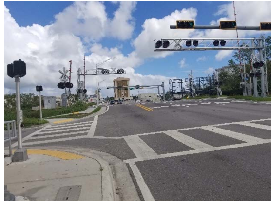
5. NE 4 th Avenue @ 79 th Street intersection facing east
