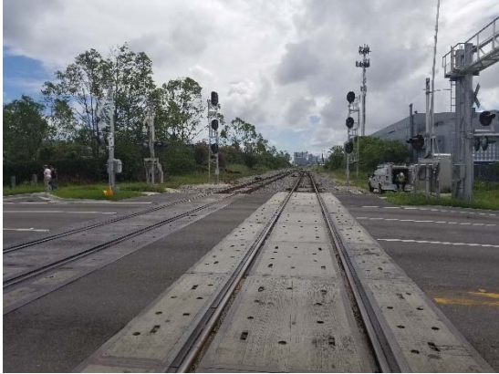
1. Railway facing north
