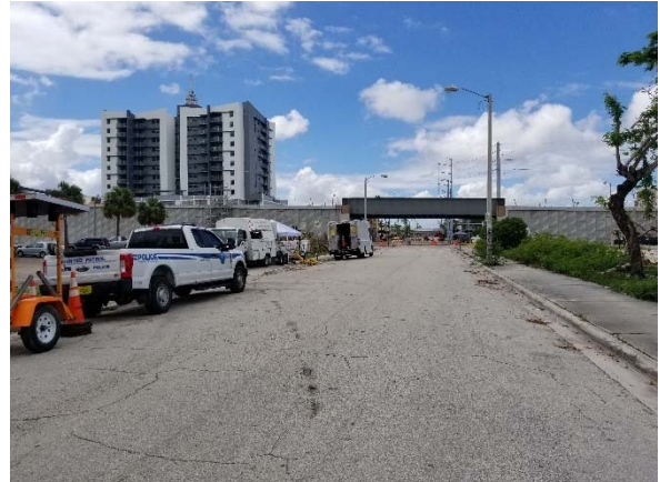
4. NE 11 th Street facing west. Notice the above grade rail crossing.
