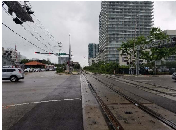
4. NE 36 th Street tracks facing south
