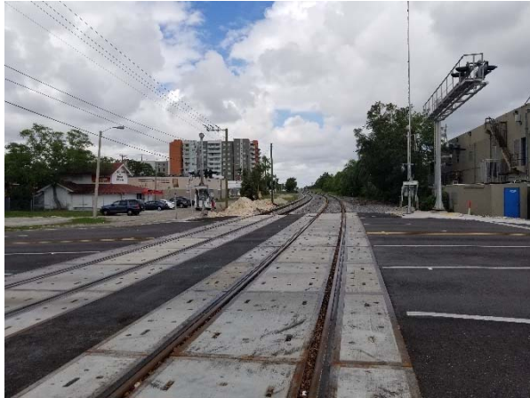
1. Railway facing north
