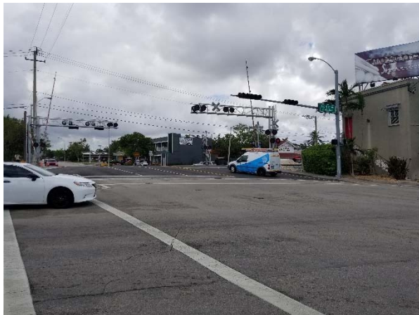
2. NE 55 th Street @ Federal Hwy intersection facing west
