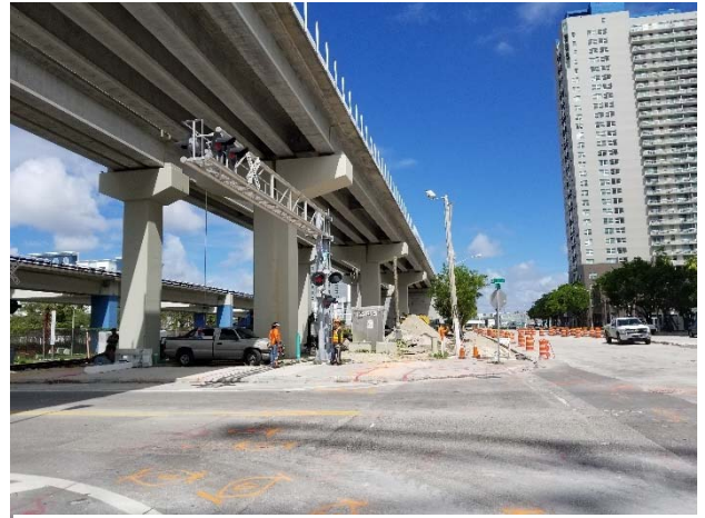
10. Brightline / Tri-Rail Coastal Link above grade connection to downtown Miami.
