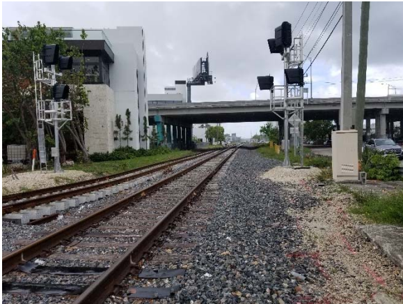
1. NE 36 th Street tracks facing north
