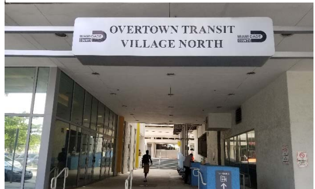
6. Overtown Transit Village adjacent to Metrorail station. The building includes headquarters for Miami-Dade Department of Transportation and Public Works.
