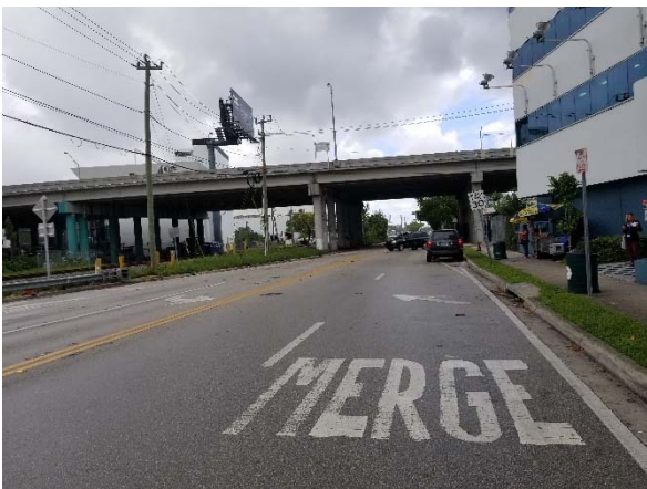
3. Federal Hwy facing north
