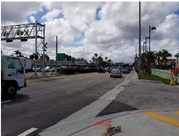
3. NE 163 rd Street facing west
