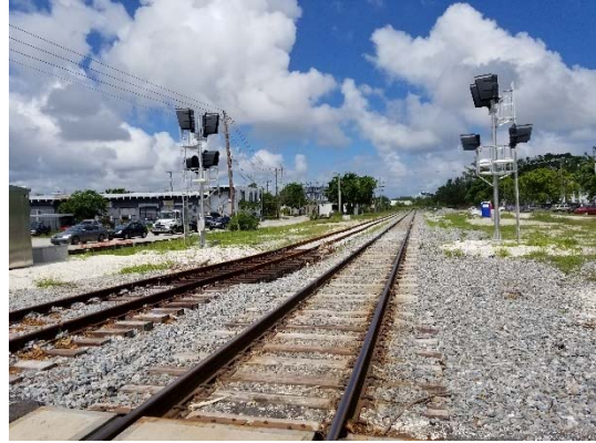
4. Existing rail line facing north
