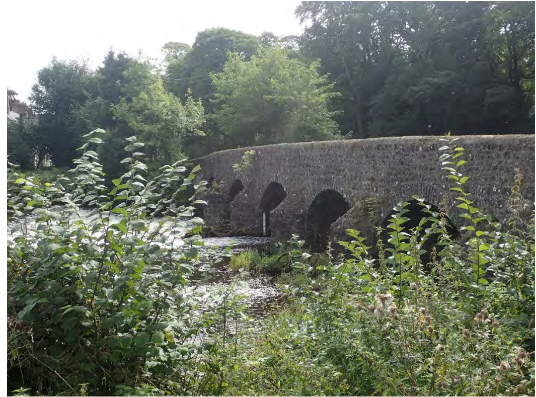
Stone bridge over Kells Water – view from Grove Road/Shankbridge Road junction
