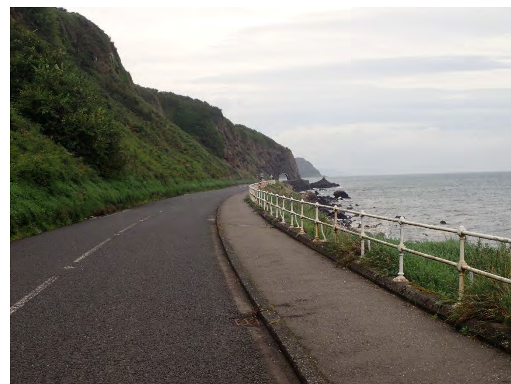
View along A2 Coast Road towards the Black Arch
