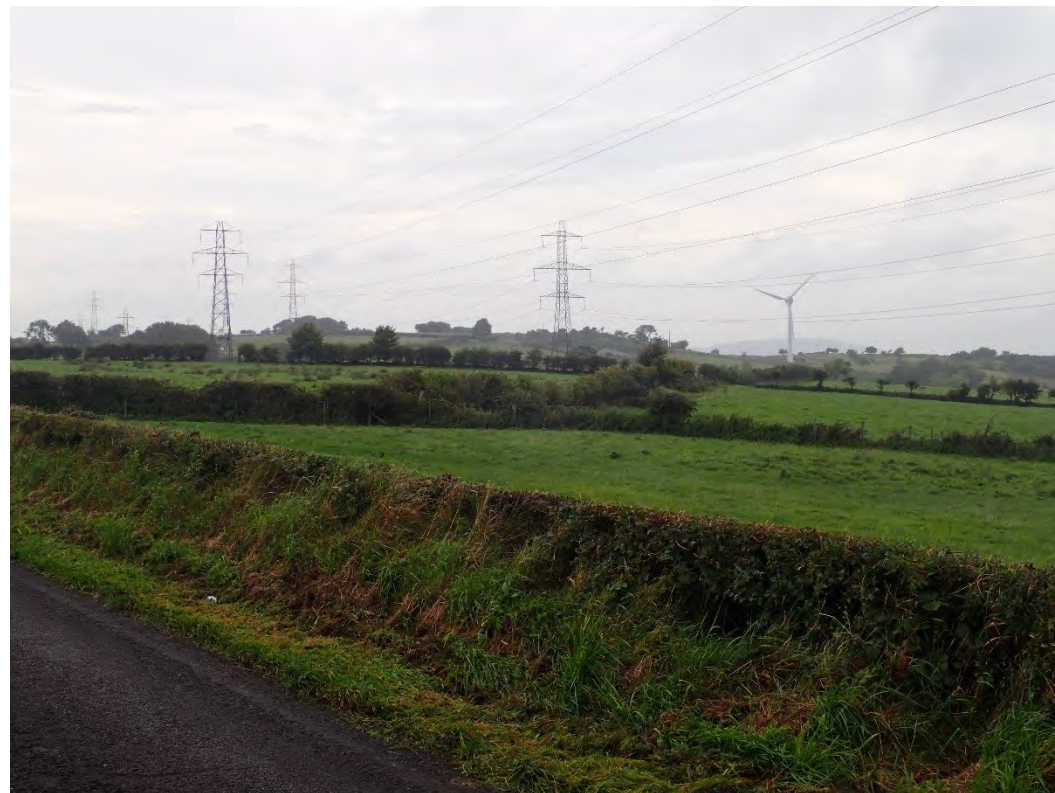
Pylons and wind turbine – viewed from Upper Carneal Road
