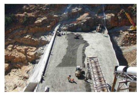
Figure 0-5 Example of RCC Dam Construction
