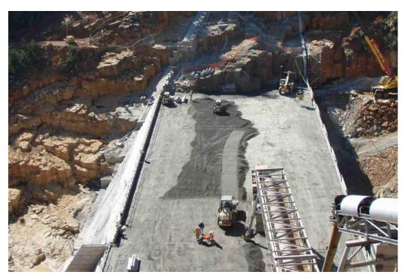
Figure 2-5 Typical RCC dam construction with concrete conveyor
