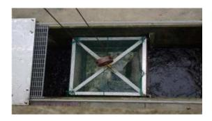
Figure 11-3 shows the trap system with ramp leading to a holding tank and piped water supply installed at Waitaki Dam, New Zealand. The ramp can be lined with bristles, gravel or a drainage
