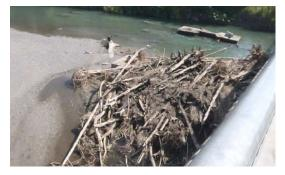
8D. Accumulation of wood at the bridge pile
