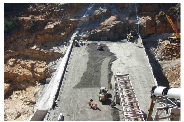
Figure 2-4 Typical RCC dam construction with concrete conveyor
