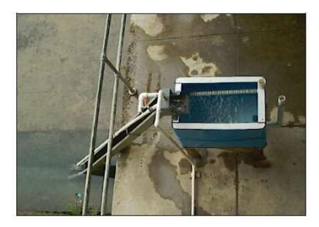
Figure 17: Example of trap installation at dam.
