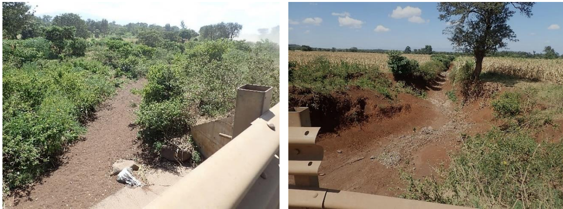
Figure 4-4 Drainage line viewed upstream (below left) and downstream (below right)
