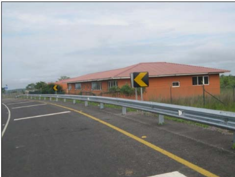
Photo 4.105: The abandoned health center in Ngola Ndala.
