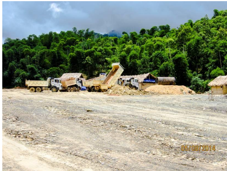
A landfill along HW 15
