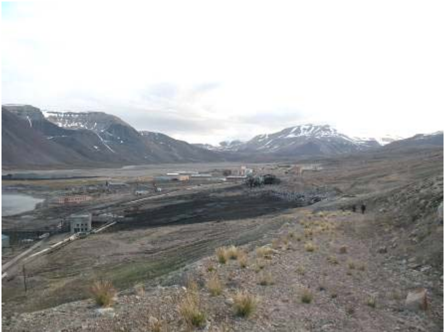
Fig. 3.1.26. The way back by the upper road on the slope of Mt. Pyramiden. Photo by O.Belkina
