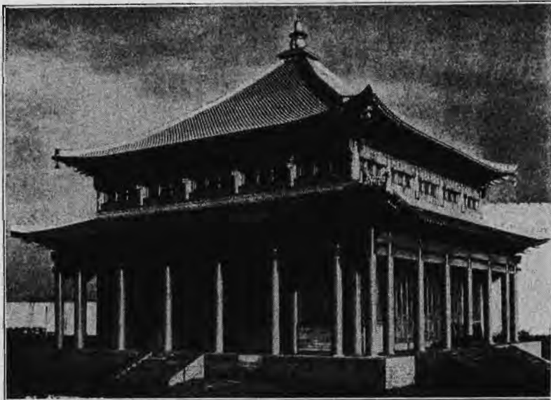
Exterior of The Golden Pavilion
