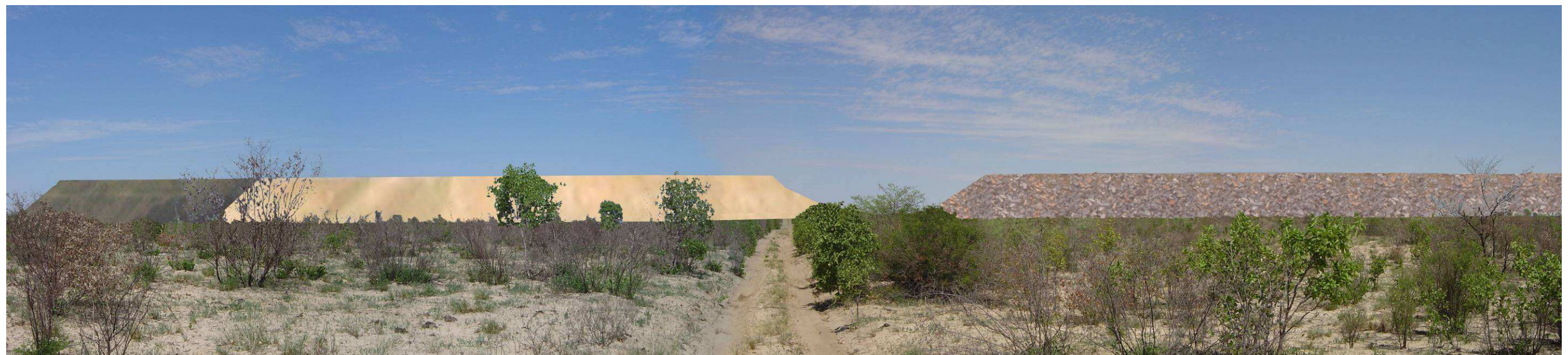
Figure 56: Photograph Showing a View Towards the Gope Project Site Showing the Sand Dump, WRD as well as the TMF from 5km (the Simulation Assumes NO Vegetation Cover on the Mine Residue Dumps).
