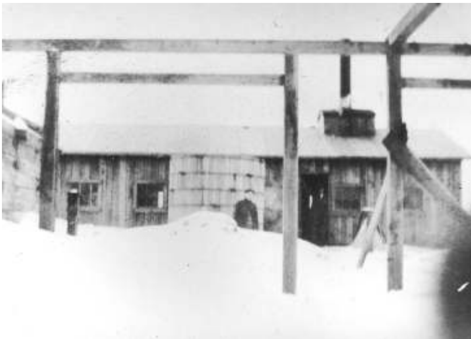
The Choate Mine water tank and stack in the winter of 1918.
