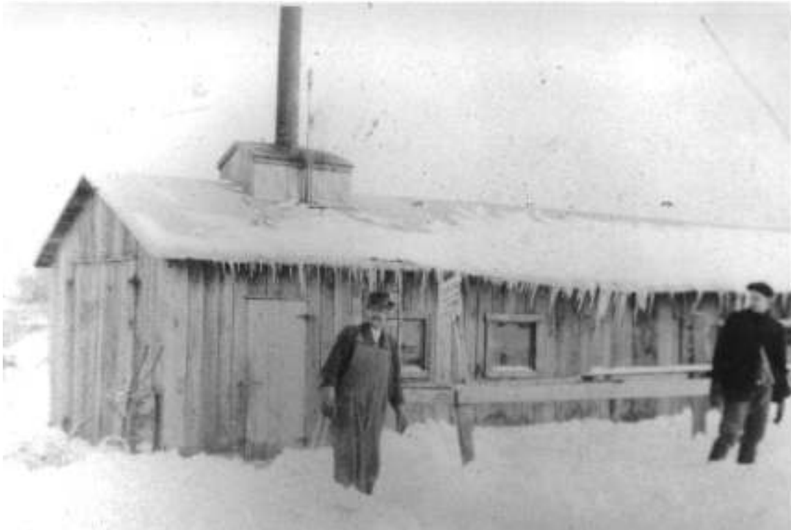
The completed Choate Mine building in the winter of 1918.
