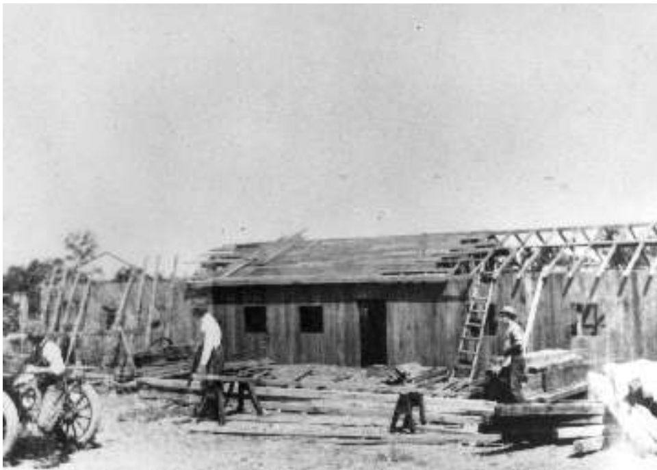
The Choate Mine building under construction in the fall of 1917.
