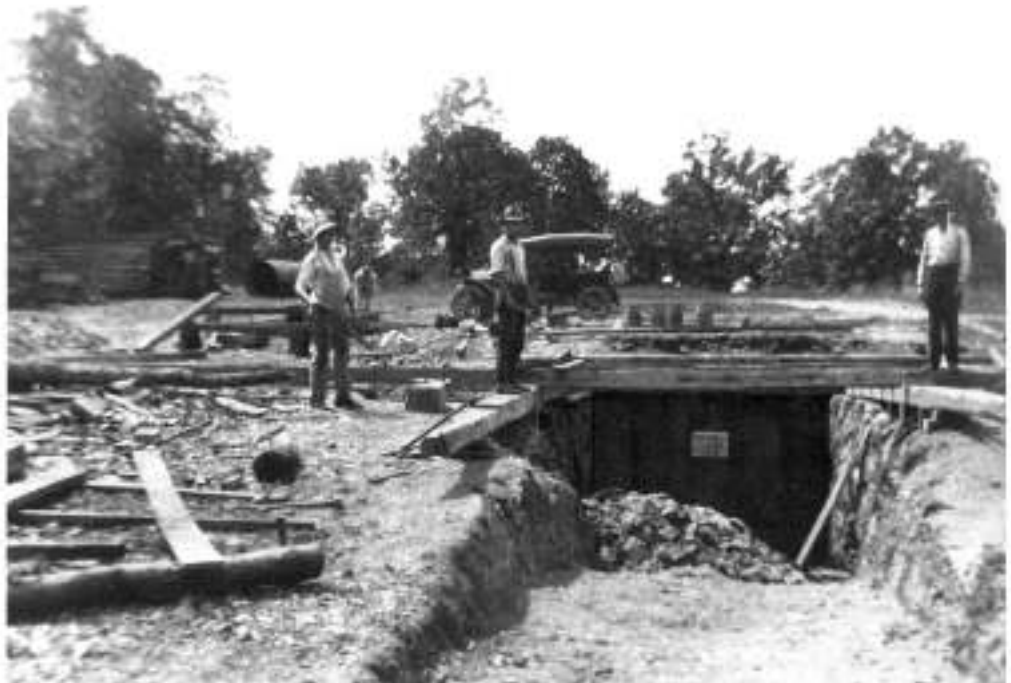
Outfitting the Choate Mine for production during World War I. The automobile in the photo is John Buxton's 1911 Stoddard-Dayton. Also note the stacks of lumber, apparent boiler, and nail kegs in the photo.
