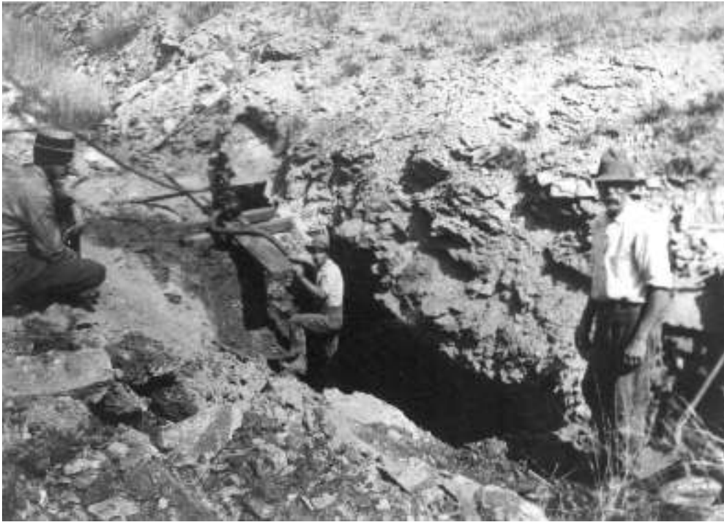
Preparing the Choate Mine for production during World War I; dewatering with a pump in the summer of 1917. (All 1917 vintage photographs were taken by Ralph Ewing "Ted" Buxton, nephew of John Buxton, Jr., and are provided courtesy of Jane Buxton Cameron and Colby Rucker, grandniece and grandnephew of John Buxton, respectively.)
