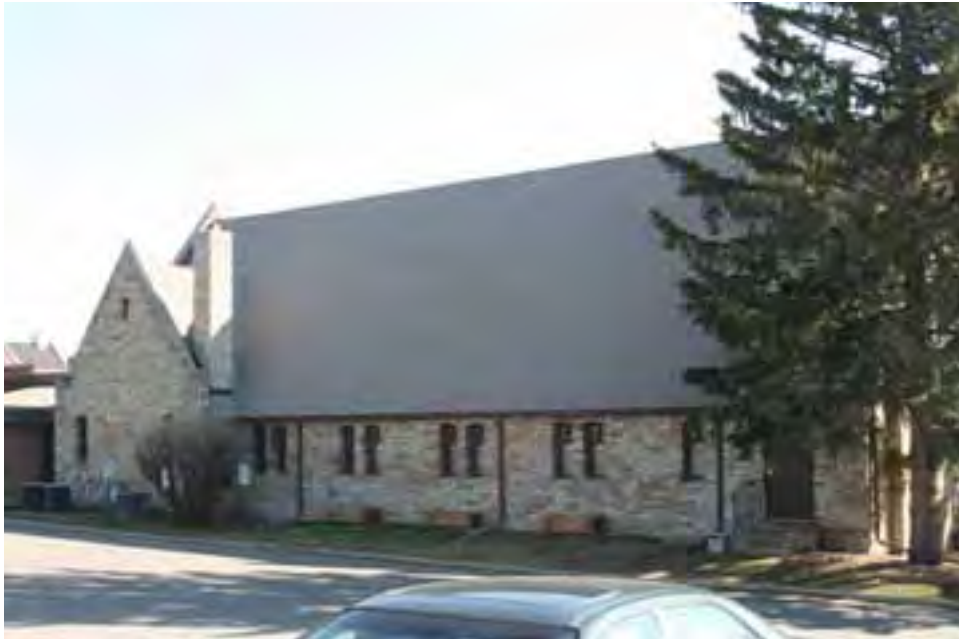
Figure 69. Union Congregational Church rear (west) elevation, view facing northeast.
