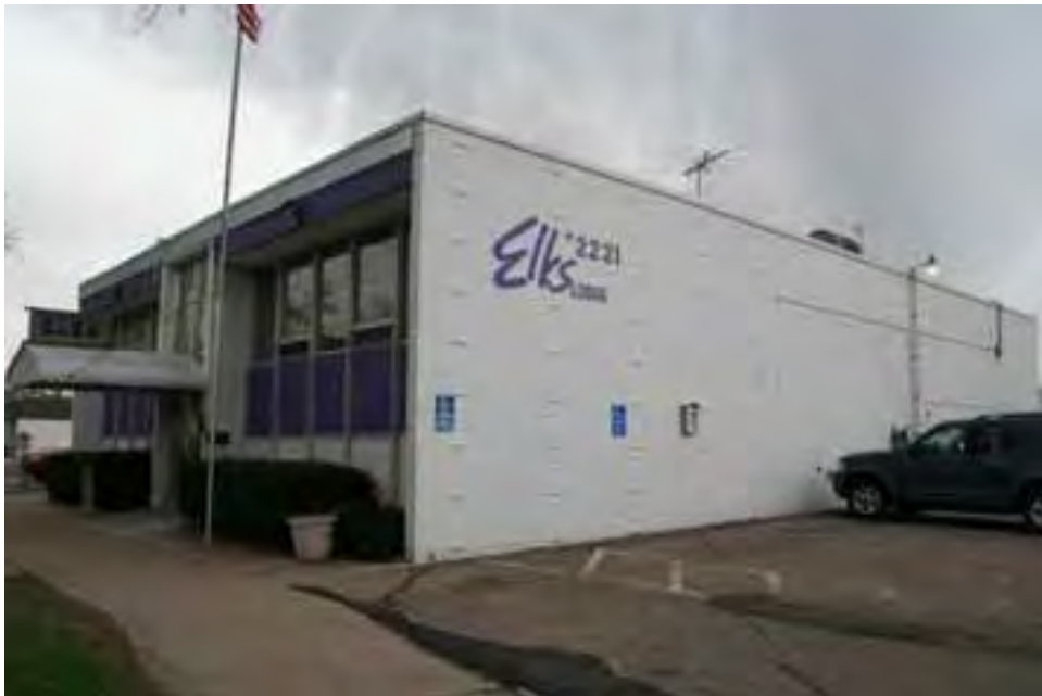
Figure 48. Oblique view of east and north elevations, view facing southwest.
