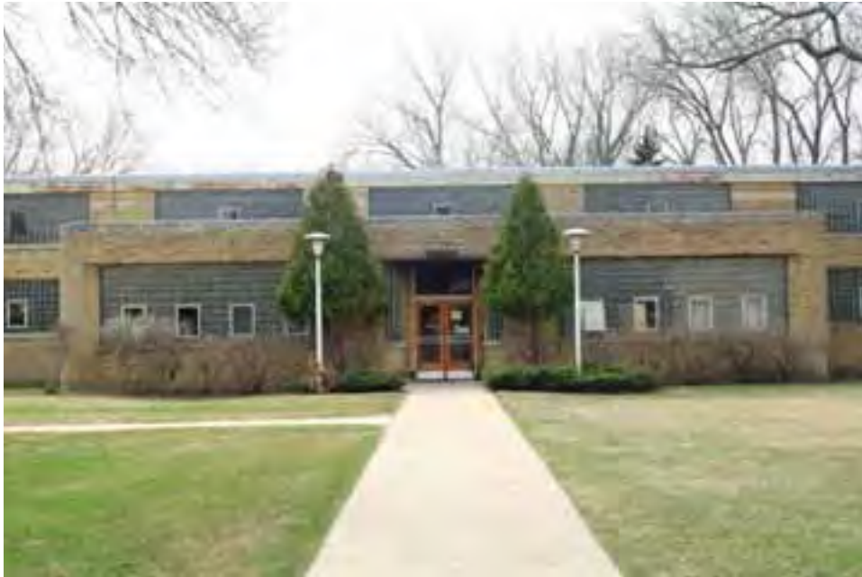
Figure 62. Woodmark Industries Building office bay, view facing south.
