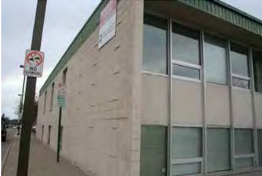
Figure 51. Oblique view of south and east elevations, view facing northwest.
