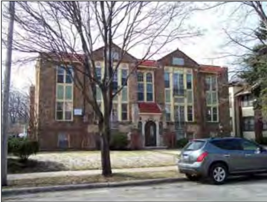
2806 Xerxes Avenue South
