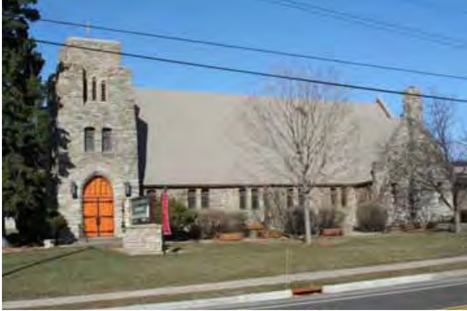
Figure 68. Union Congregational Church front (east) elevation, view facing west.
