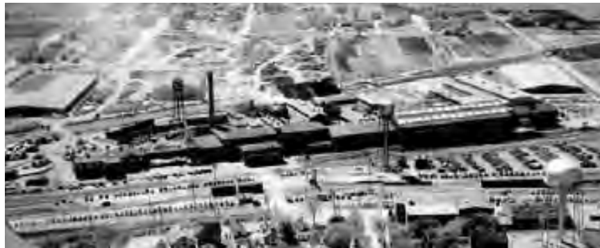
Figure 5. Minneapolis Moline complex in Hopkins, c.1925 (Minnesota Historical Society, Negative 49295).
