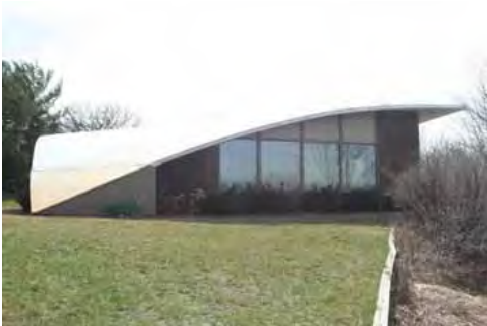
Figure 16. Northwest elevation, view facing southeast.
