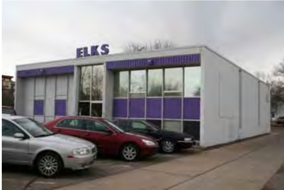
Figure 49. Oblique view of west and south elevations, view facing northeast.
