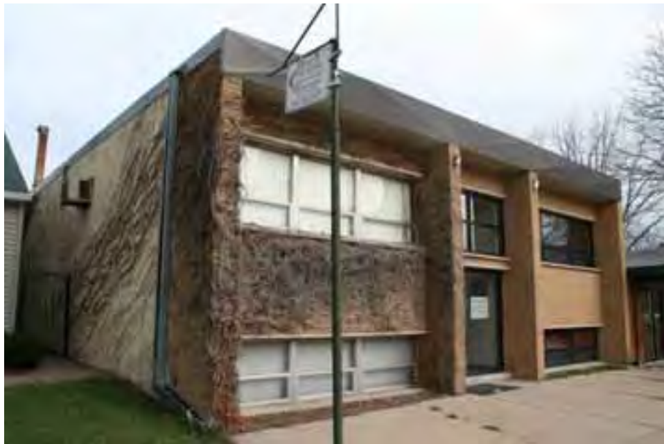
Figure 53. Oblique view of west (primary) and north elevations, view looking southeast.
