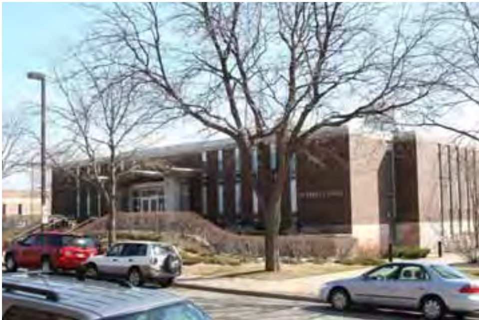
Figure 23. North facade of Hopkins City Hall, view facing southeast.
