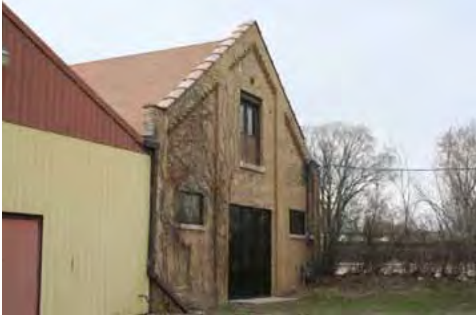
Figure 17. Original portion of the building, view facing northwest.
