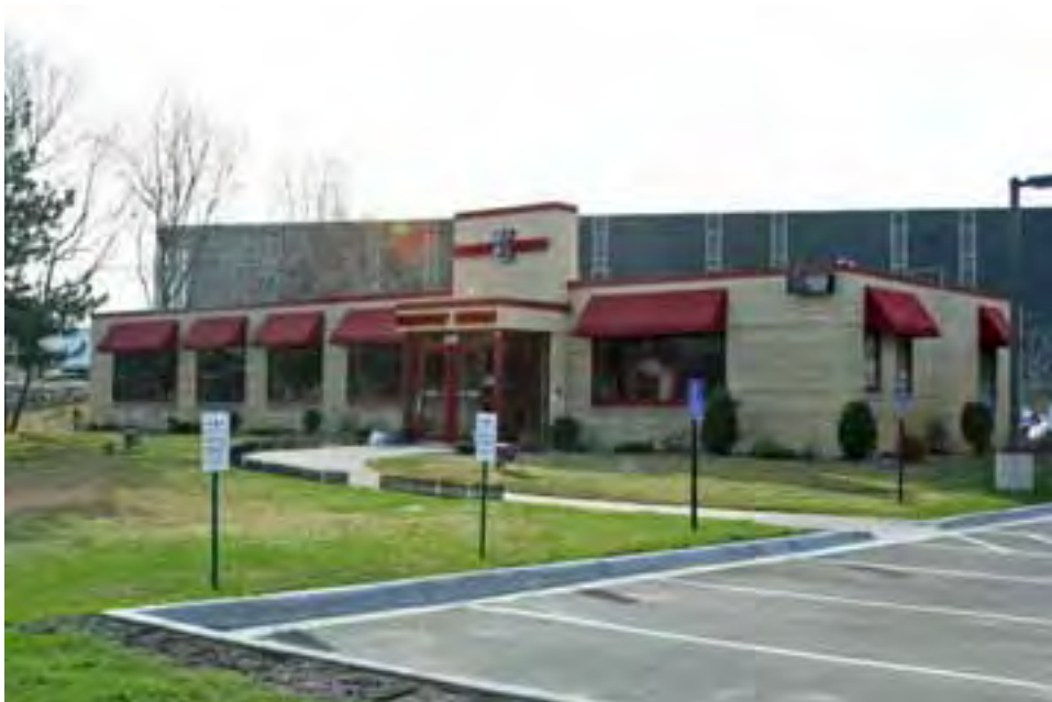
Figure 77. Building #4 facade and west elevation, the structure was built in 1950 and added to the Northland Aluminum building inventory in 2006, view facing southeast.
