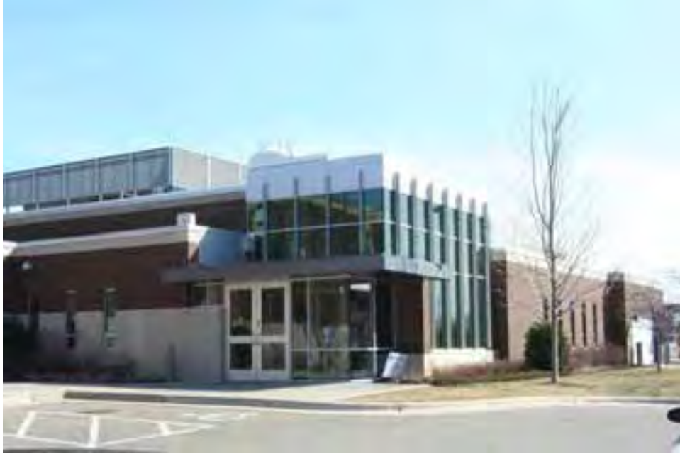
Figure 26. 2003 addition to the west elevation, view facing southeast.
