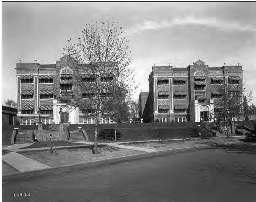
Calhoun Beach Apartments shortly after completion, 1925 Hibbard Studio photograph—Minnesota Historical Society Collections
