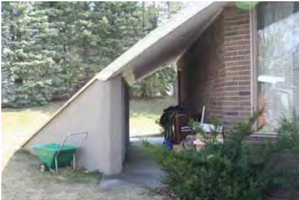
Figure 14. Detail view of the concrete anchors.
