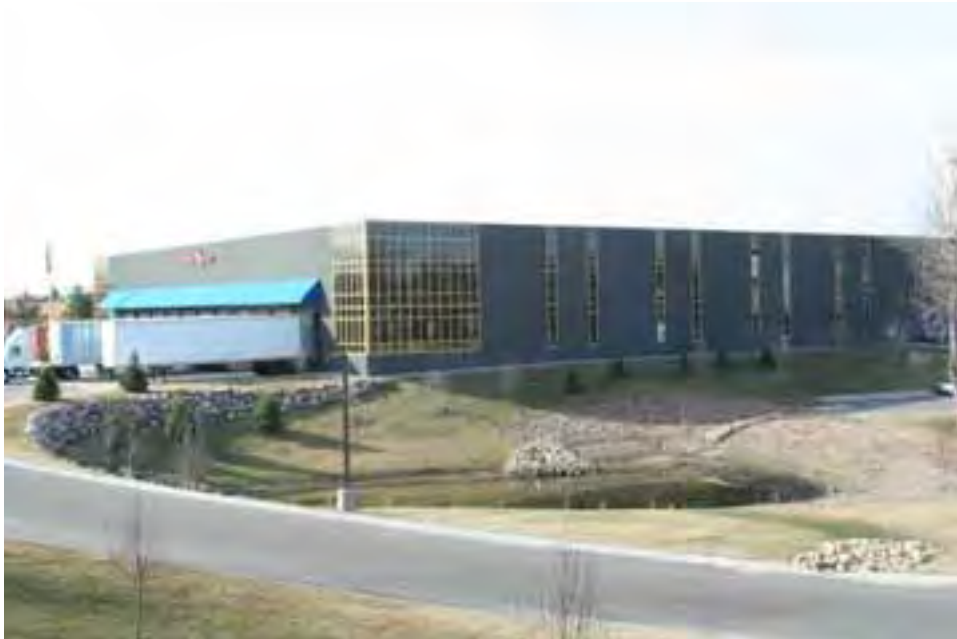
Figure 79. Northeastern elevation of Building #7 showing both glass corners and loading docks, view facing southwest.
