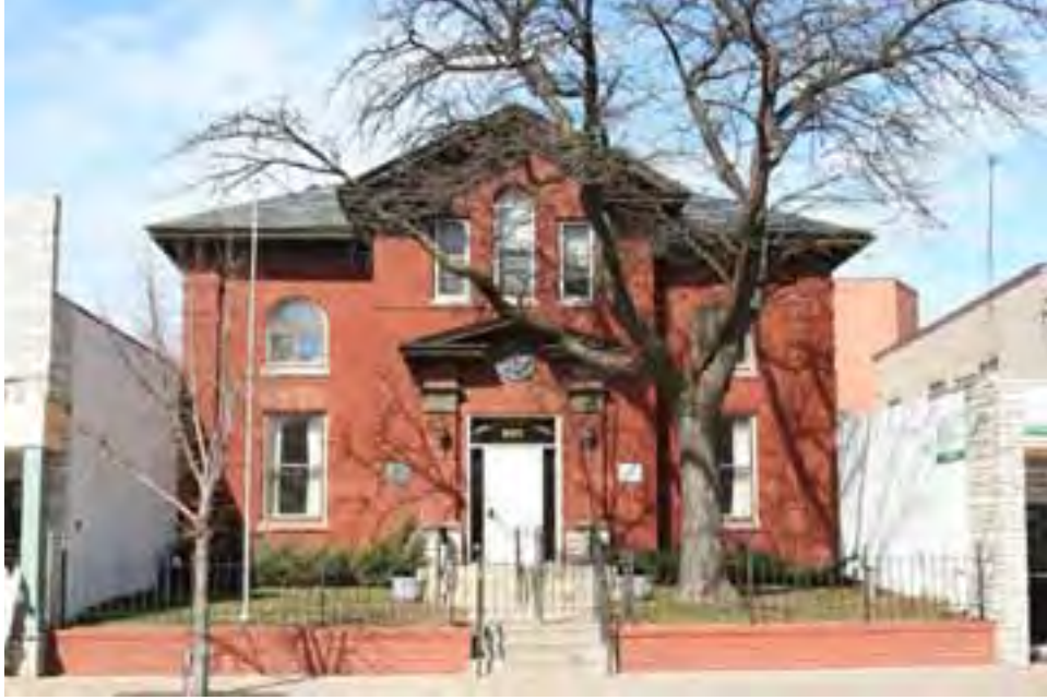
Figure 35. The 1902 Albert Pike Masonic Lodge located at 907 Mainstreet, view facing north.
