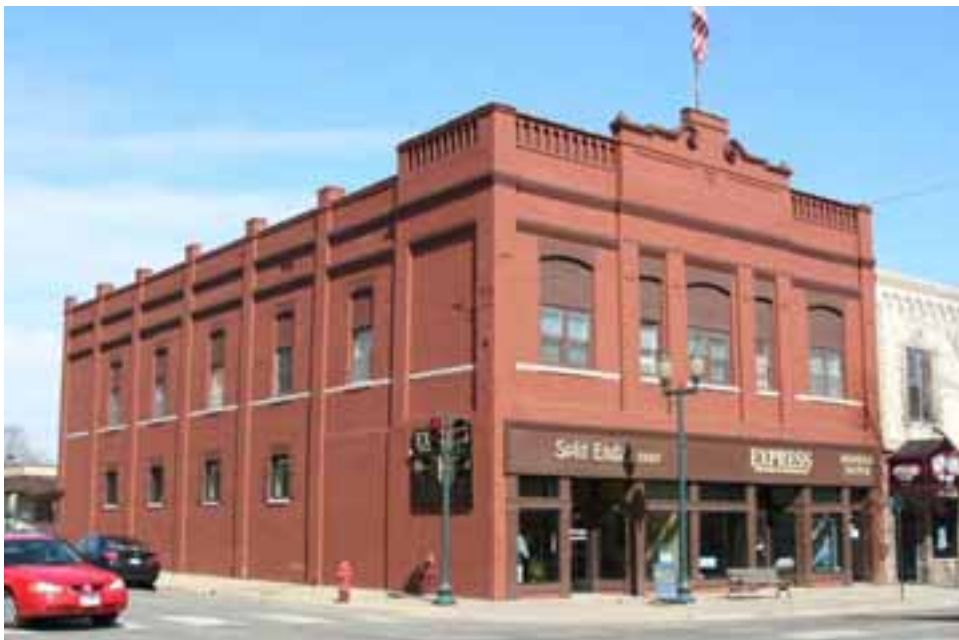
Figure 34. The 1903 IOOF building located at 823 Mainstreet, view facing northeast.
