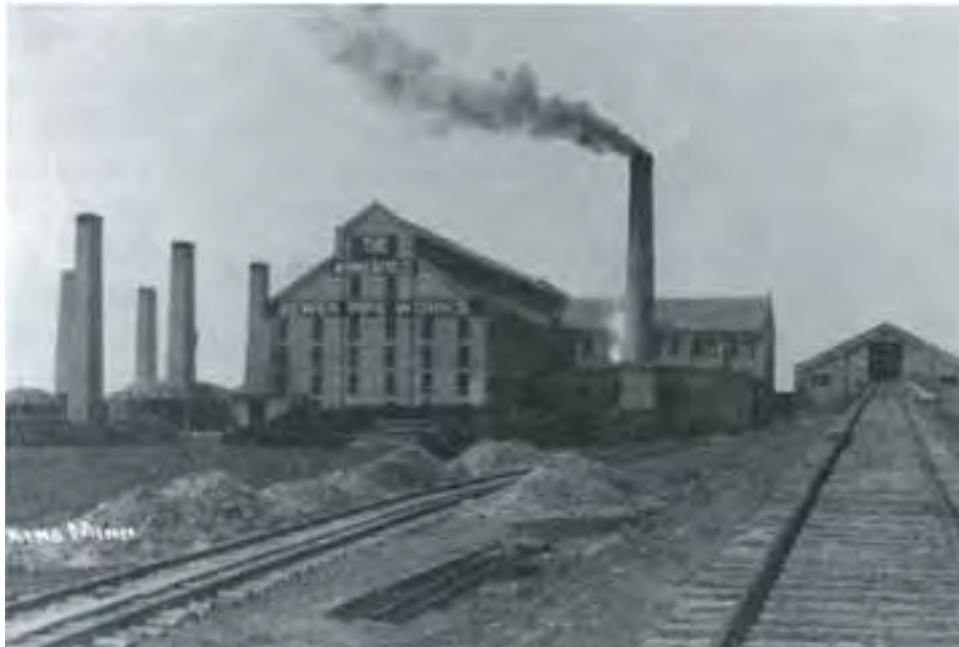
Figure 21. Red Wing Sewer Pipe Company. Subject building is visible on right (Hopkins Through the Years, 59).
