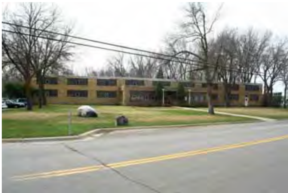
Figure 61. Woodmark Industries Building, view facing southwest.
