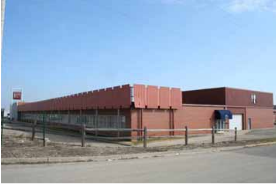
Figure 43. Former Minneapolis Moline building, front (north elevation), view facing southeast.
