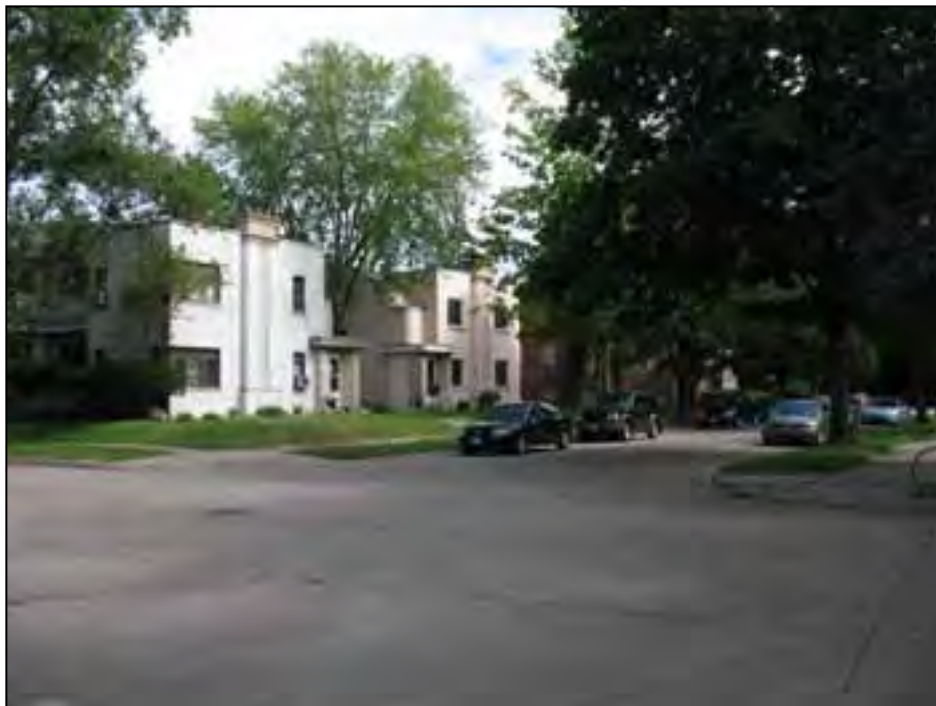
Street view, 2800 Block of Xerxes Avenue South
