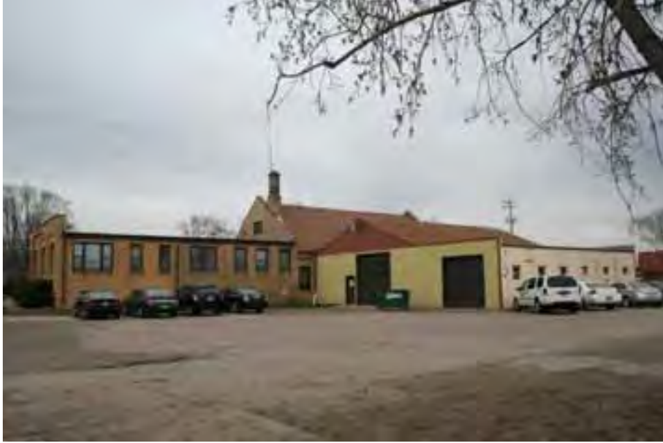
Figure 19. Original brick structure and additions, view facing northeast.
