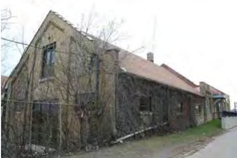
Figure 18. Original building and c.1950 brick addition, view facing southwest.
