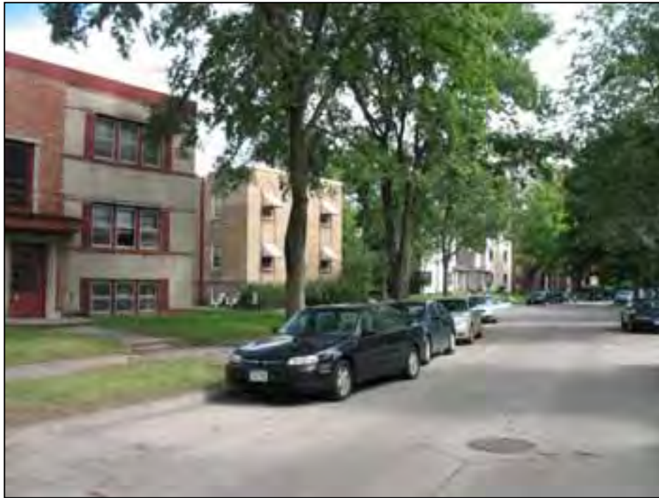
Street view, 2700 Block of Xerxes Avenue South
