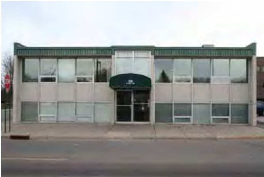
Figure 50. East (primary) facade, view facing west.
