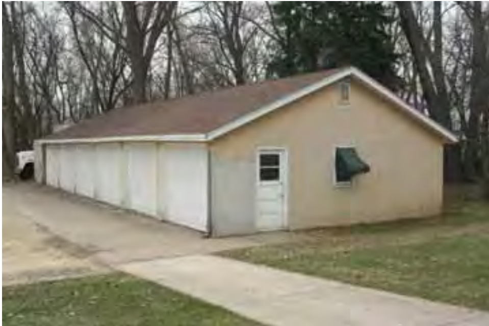
Figure 65. Woodmark Industries Building, garage building at rear of property, view facing southwest.
