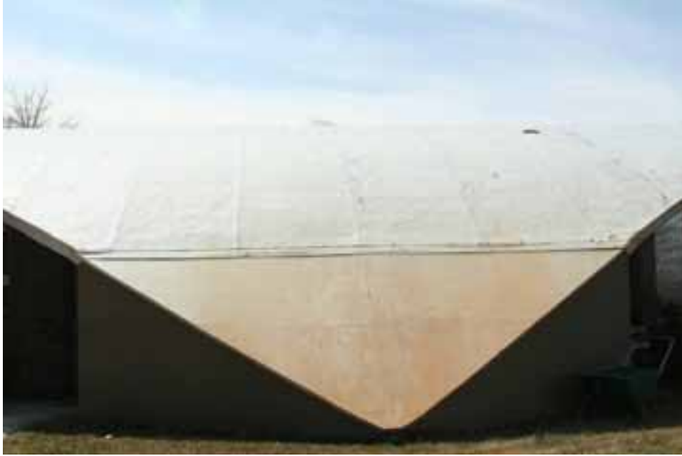
Figure 15. Detail view of the roofing materials.
