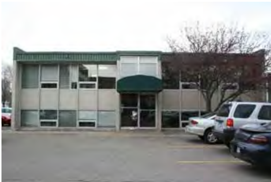
Figure 52. West elevation, view facing east.
