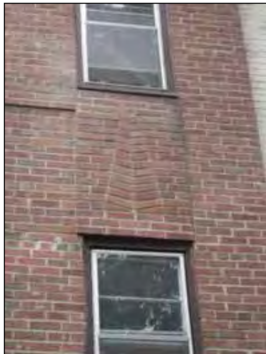
Detail of brickwork on apartment buildings
