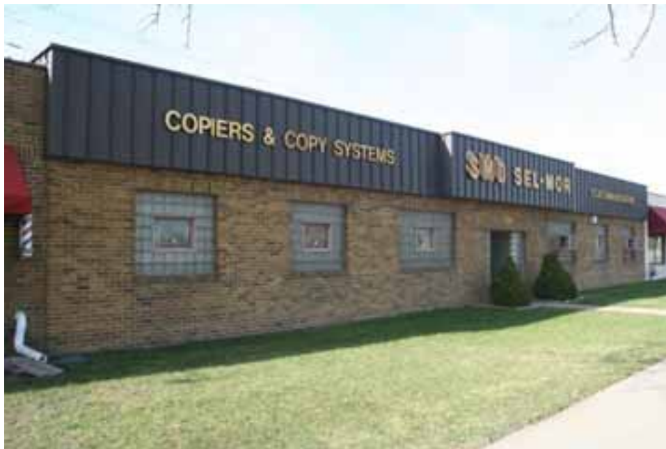
Figure 66. SMD Sel-Mor building, 6520 West Lake Street, Minneapolis, view facing north.
