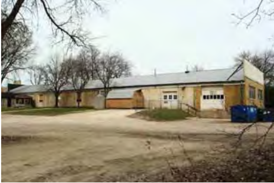
Figure 64. Woodmark Industries Building, south and east elevations, view facing northwest.
