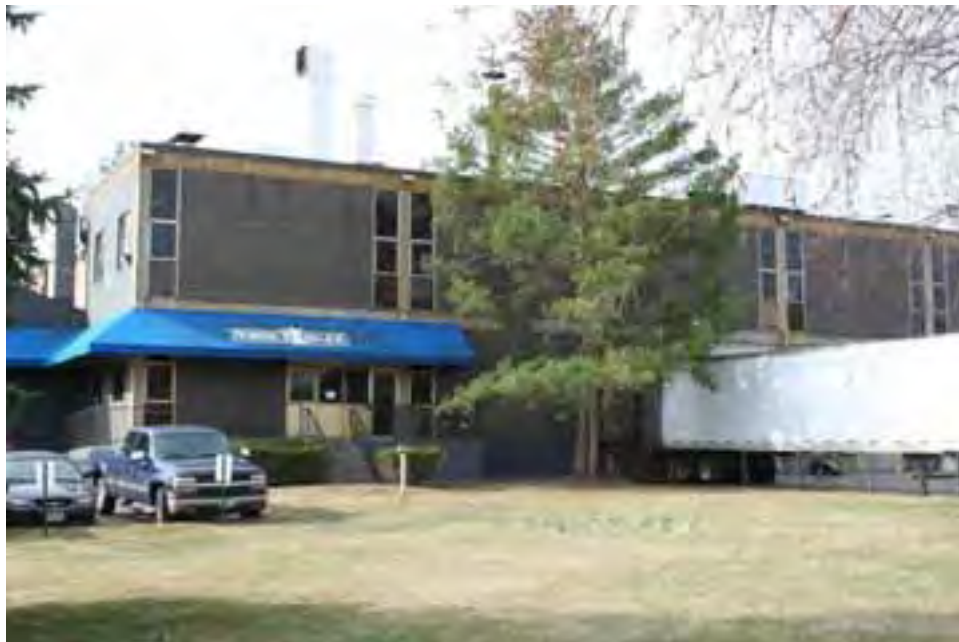
Figure 75. Northeast corner of Building #1, the prestressed concrete panels were added as part of the 1968 building addition, view facing southwest.
