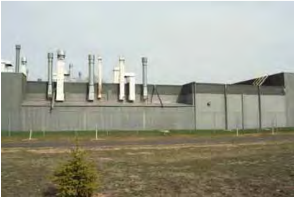
Figure 76. Rear elevation of Buildings #2 and #3, view facing north.
