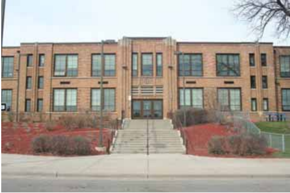
Figure 56. St. Louis Park High School, 1937 building, front (south) facade, view facing north.
