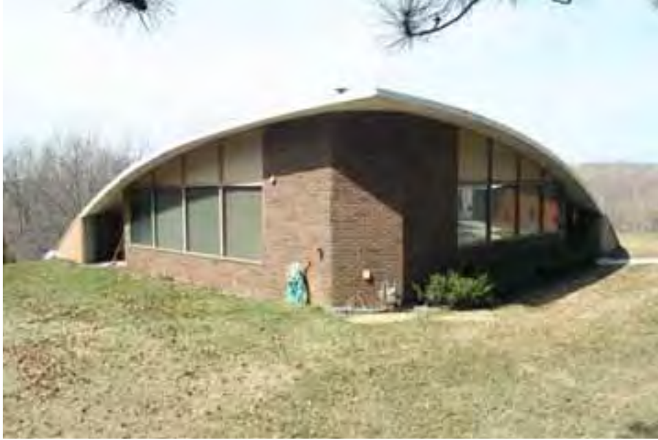
Figure 13. Note how the north and south sides of the roof are pinned to the ground while the east elevation is allowed to extend, view facing southwest.
