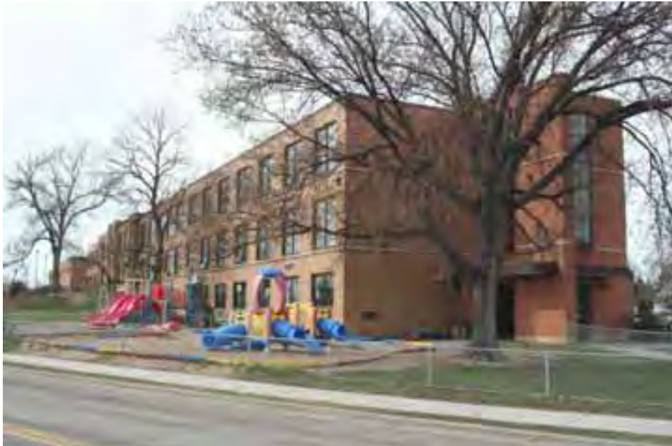
Figure 57. St. Louis Park High School, 1937 building with additions on front (south) and side (east) elevations, view facing northwest.
