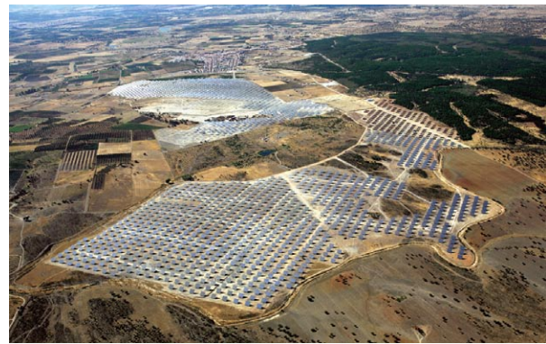
Solar photovoltaic generation facility (Moura)
