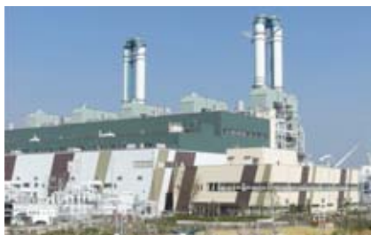
The Kansai Electric Power Co., Inc.'s Sakaikou Power Station was completed in September 2010. This LNG-fired plant with an output of 2 million kW, achieves generating efficiency of 58%, one of the highest levels in the world.
