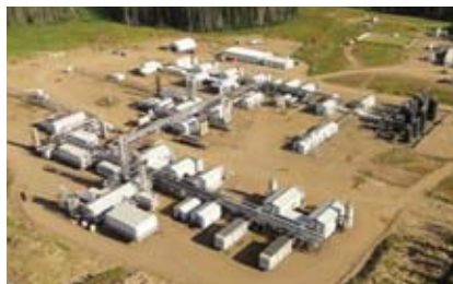
A gas treatment plant at the shale gas development in British Columbia, Canada
