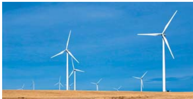
U.S.-based Diamond Generating Corporation, a wholly owned MC subsidiary, owns the Goshen II wind farm in the state of Idaho.
