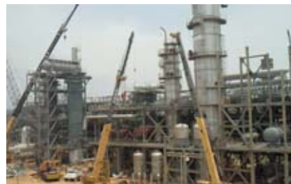
METOR is a joint venture between MC, Venezuelan state-owned company Pequiven, Mitsubishi Gas Chemical Company, Inc. and others. In the year ended March 2011, METOR completed construction of an 850,000 ton/year second facility adjoining an existing plant that is capable of producing 750,000 tons of methanol a year. Commercial operations at the new facility began in August 2010.
