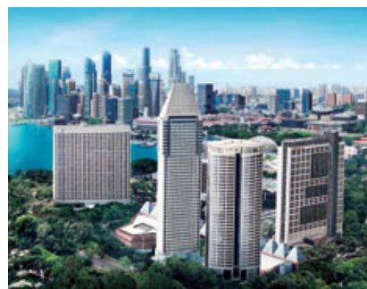
MC has established a subsidiary in Singapore for coordinating its mineral resources trading business. The company is tenanted the building second from the right.
