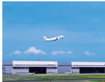
Pictured is the IIF HANEDA Airport Maintenance Center, which is owned by Industrial & Infrastructure Fund Investment Corporation. This investment firm is managed by an MC affiliate.
