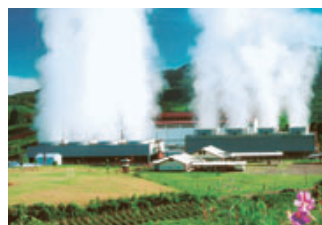
The Wayang Windu Geothermal Power Project Plant is operated by an Indonesian geothermal power generation company in which MC is an investor.
