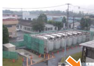
Prior to removal of private power generator
