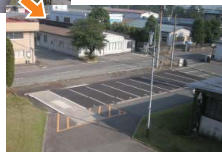
Following removal of private power generator
