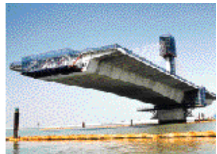
Ibigawa Bridge, part of the Daini-Meishin Highway, built using prestressed concrete produced by P.S. Corp.
