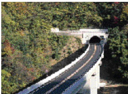
The Hachidoyama tunnel, built by Mitsubishi Construction Co., Ltd., in Matsuyama, Ehime Prefecture
