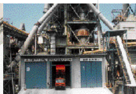
Waste recycling plant
