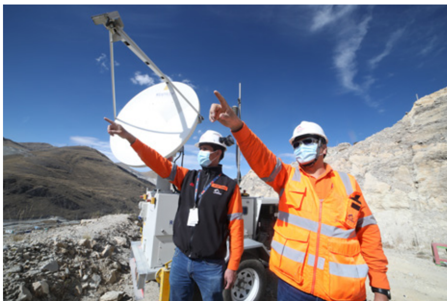
Our Technology team starts up a modern geotechnical monitoring integrated system.
