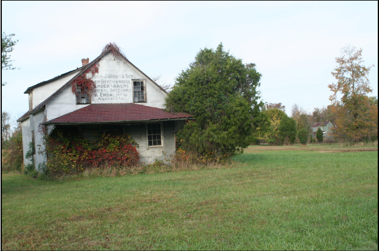
Looking northwest, James A. Cochrane Store (PG: 87B-036-17), 22609 Aquasco Road ( EHT Traceries, 2007 )
