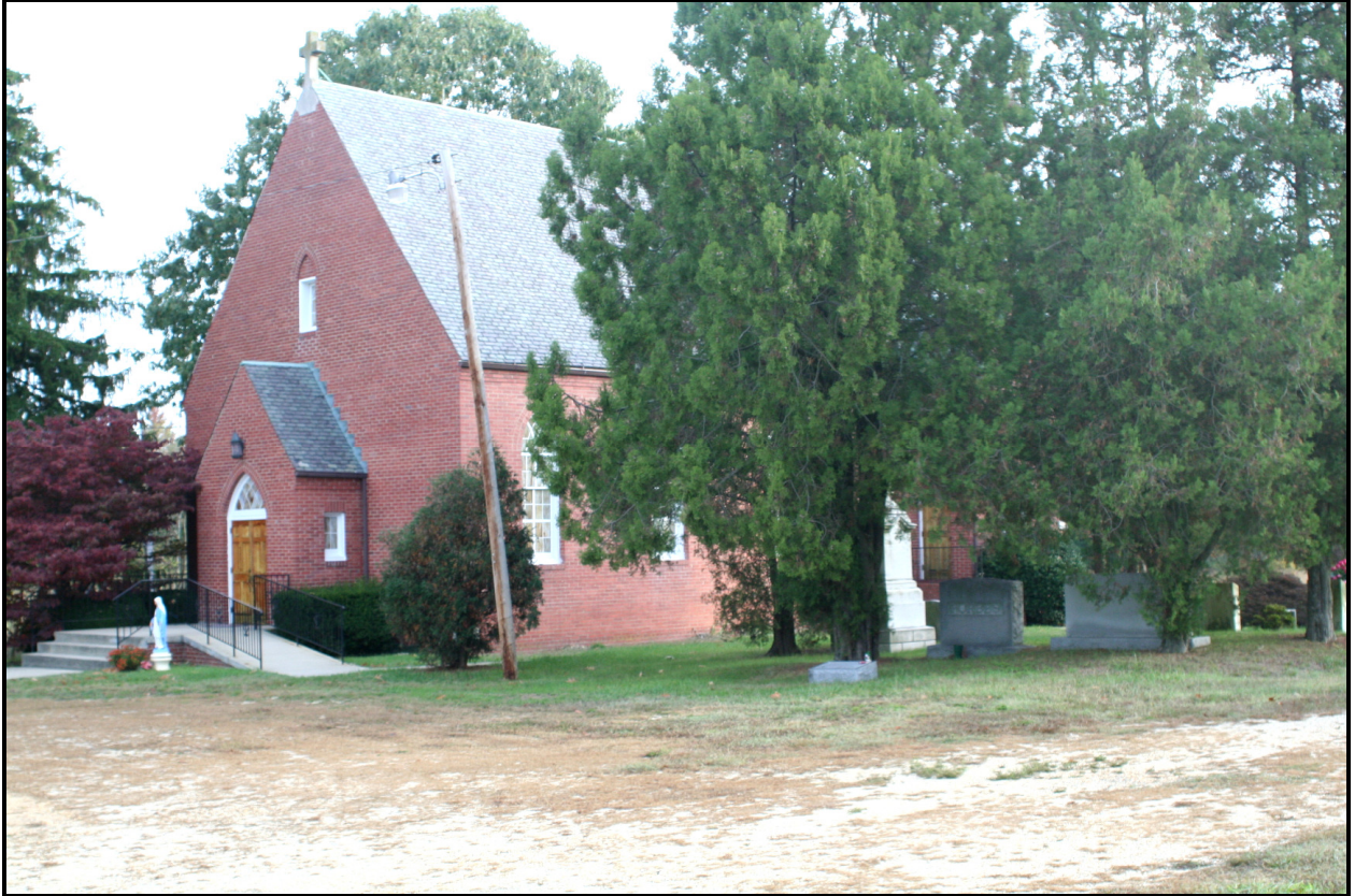
Looking northeast, St. Dominic's Catholic Church, 22300 Aquasco Road ( EHT Traceries , 2007)
