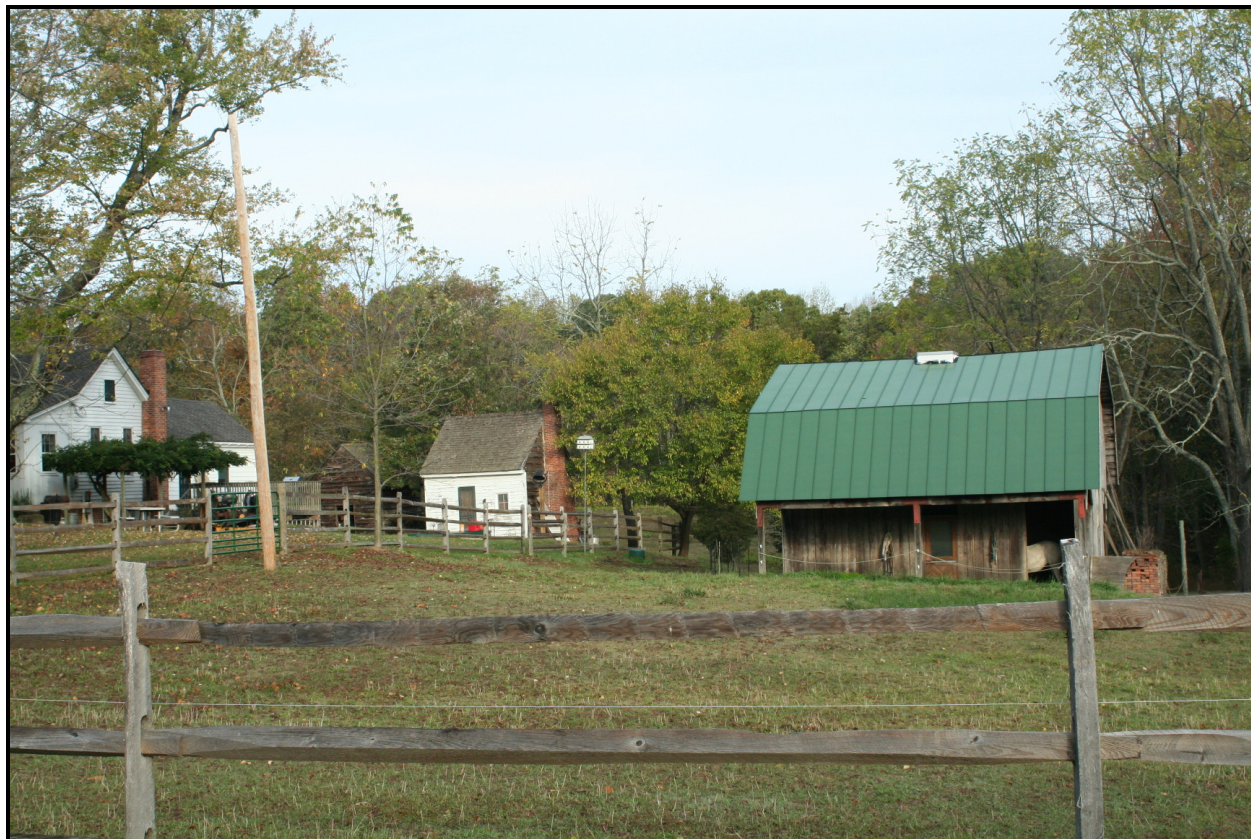
Looking north, outbuildings at J.E. Turner House (PG: 87B-036-05), 16410 St. Mary's Church Road ( EHT Traceries , 2007)
