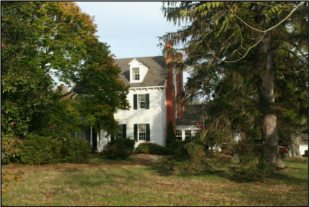
Looking north, J.E. Turner House (PG: 87B-036-05), 16410 St. Mary's Church Road ( EHT Traceries, 2007 )
