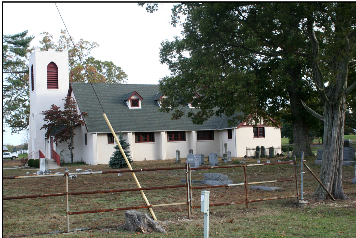
Looking northeast, St. Mary's Church and Cemetery (PG: 87B-036-08b), 22200 Aquasco Road ( EHT Traceries , 2007)
