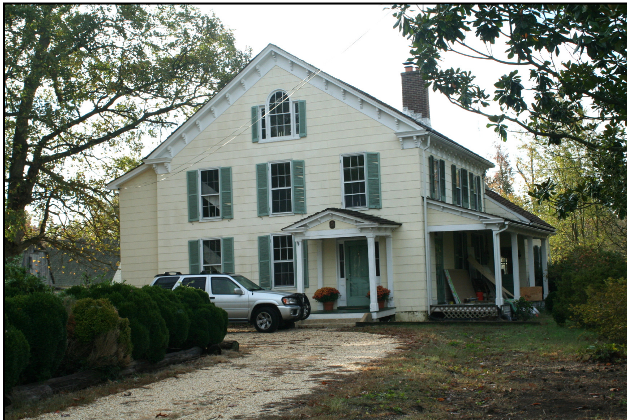
Looking south, St. Mary's Church Rectory (NR) (PG: 87B-036-08a), 16305 St. Mary's Church Road ( EHT Traceries , 2007)
