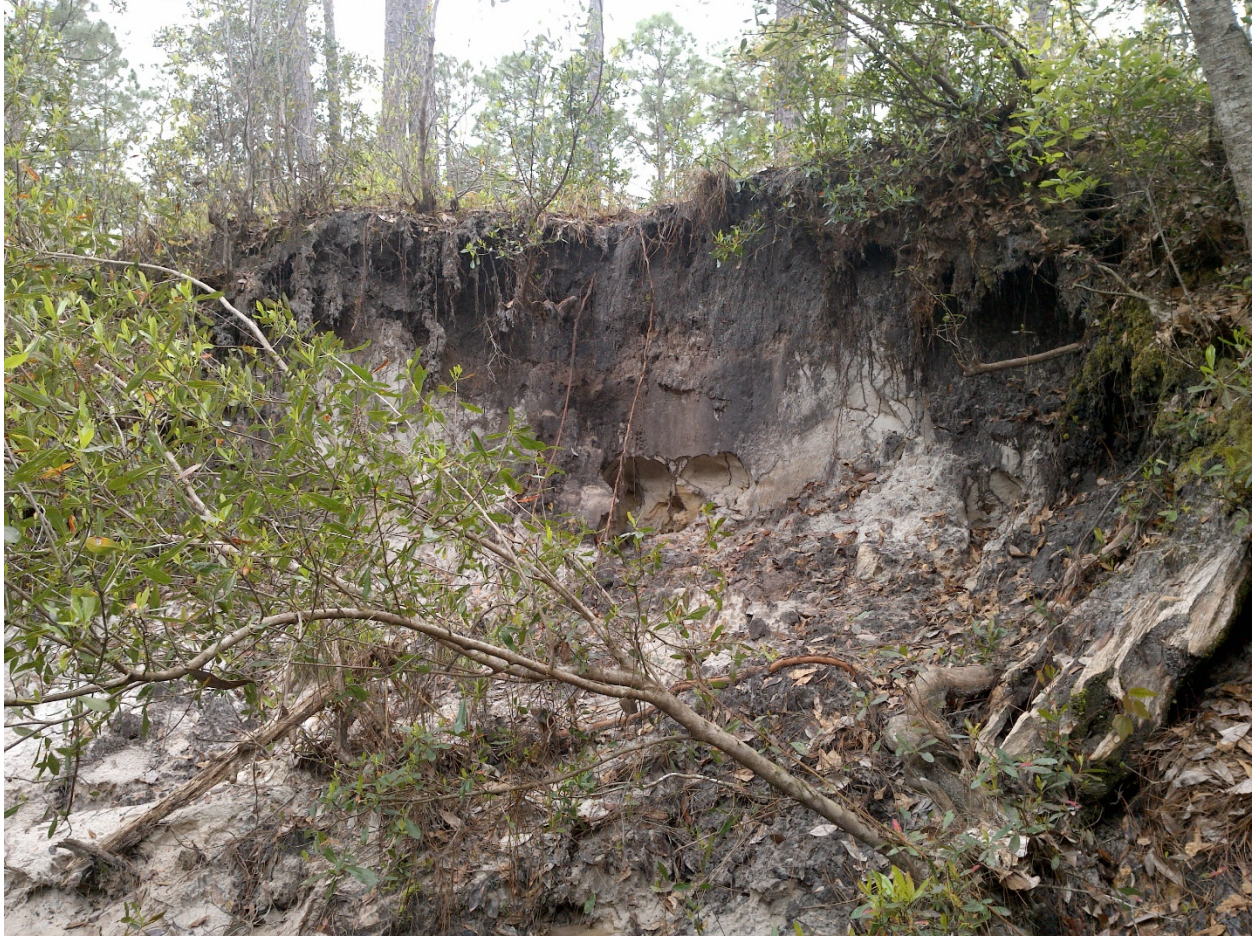
Figure 7.12 Bank Erosion Along Hammock Creek
