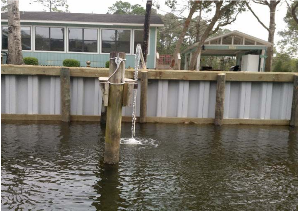
Figure 5.14 Example of Outfall Pipe Located Along Sandy Creek
