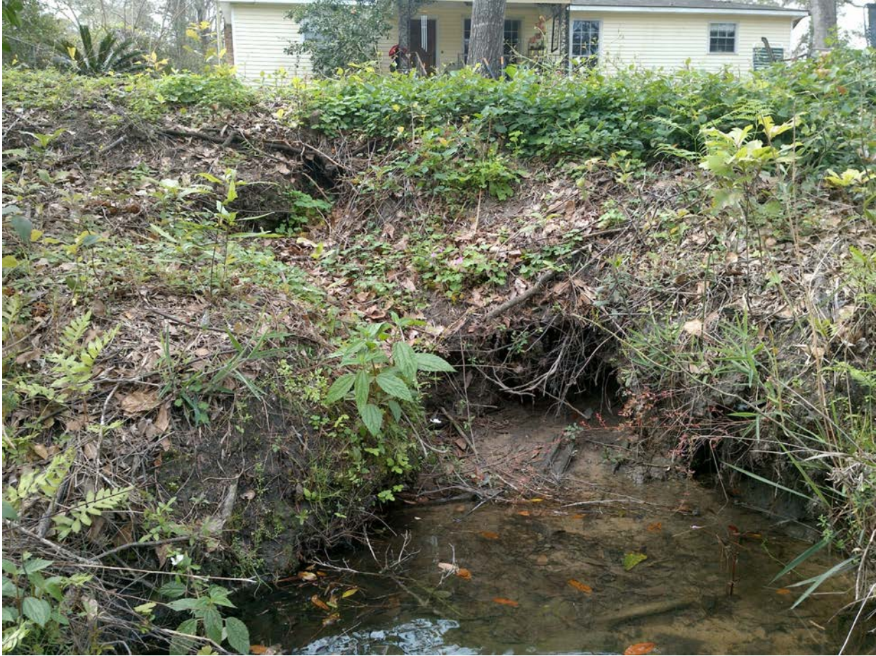
Figure 7.9 Bank Failure at Residence Along Wolf Creek
