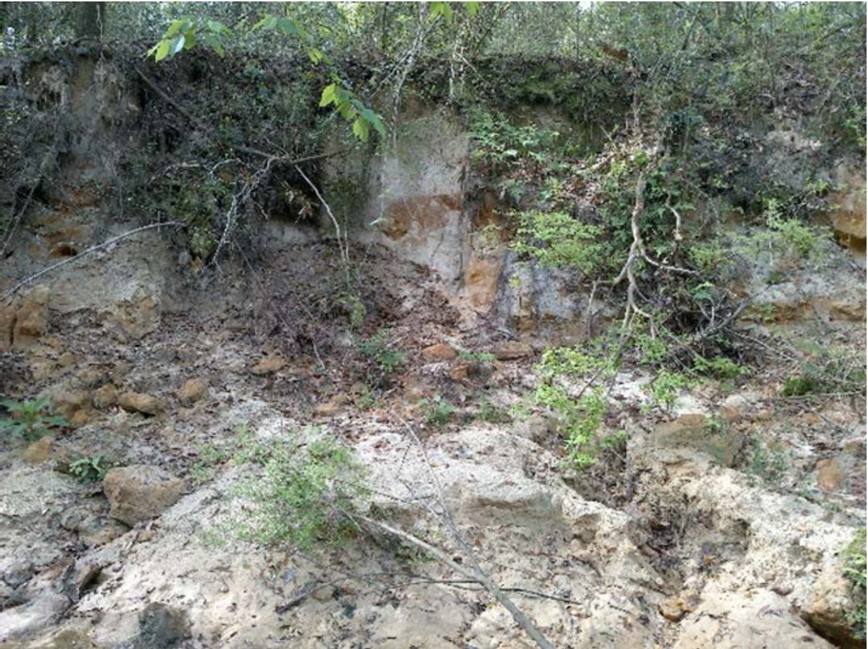
Figure 5.12 Example of Bank Instability/Sloughing Along Wolf Creek
