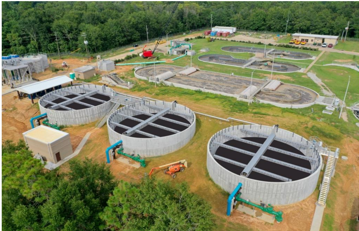
Figure 5.3 Riviera Utilities Wastewater Treatment Facility
