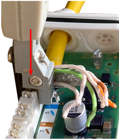
Fig. 17: Network wires connected using LSA+/Krone tool
