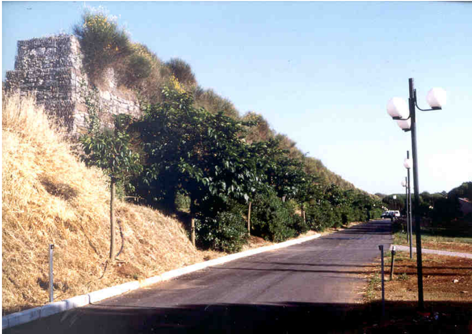
Photo 80. Noise prevention wall- a combination with vegetation
