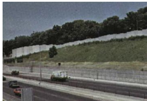
Photo 79. Excessive contrast. A darker colour would blend this barrier into the background trees
