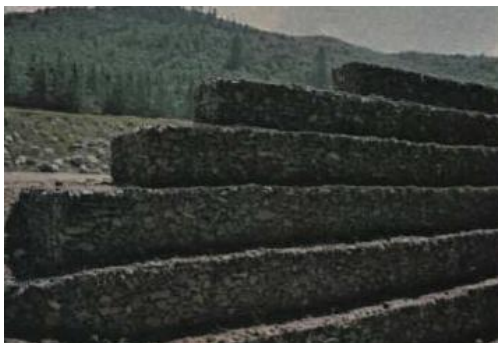
Photo 78. Gabions may be stacked in a variety of ways to construct a wall
