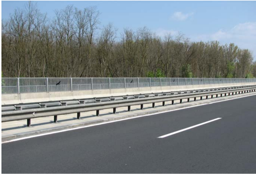
Photo 73. Protective panels for prevention of bird kills during highway operation
