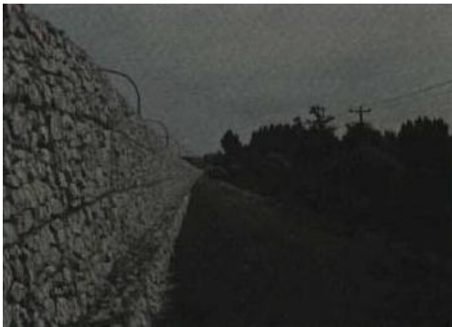
Photo 76. A gabion noise wall
