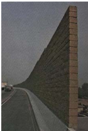
Abrupt endings on wall
