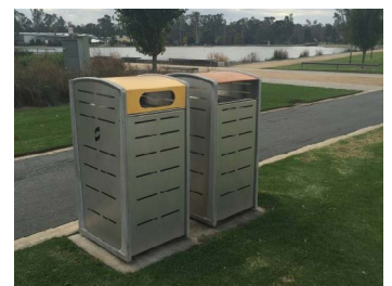
Bins on concrete slab example
