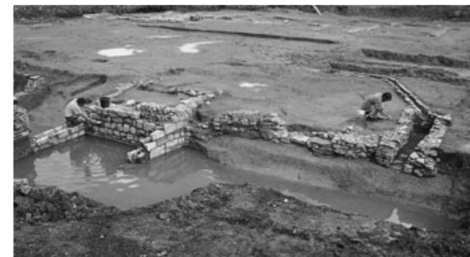
The bridge abutment, revetment and drain at the moated manor at Low Hall, Walthamstow (MoLAS)
