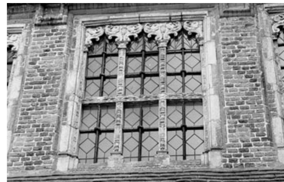
Terracotta window from Layer Marney. The mullions are from an identical mould to those used at St John Clerkenwell
