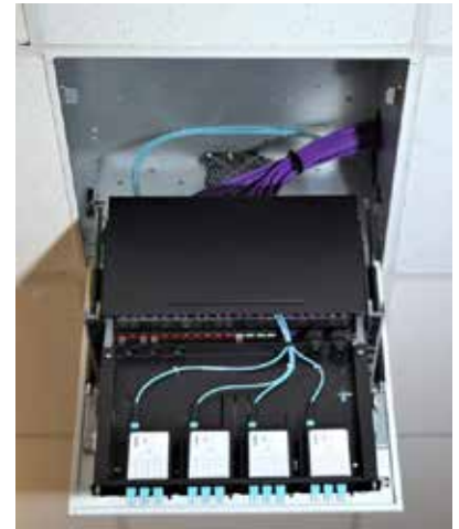
Fiber ModLink MTP/MPO installation
