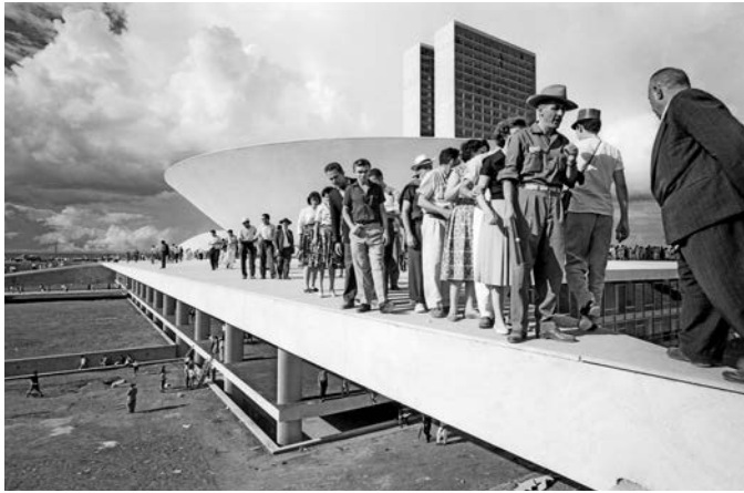
View of the roof of the National Congress on the inauguration of Brasília. April 21, 1960. Photograph by Thomaz Farkas. Instituto Moreira Salles Collection
