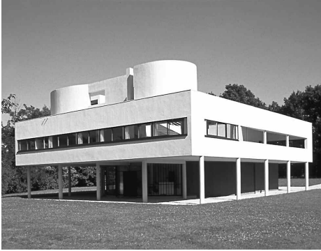
IMAGE 9: Northwest and southwest facades. 1995–99. Photo: Paul Koslowski. Fondation Le Corbusier. © 2004 Artists Rights Society (ARS), New York/ADAGP, Paris
