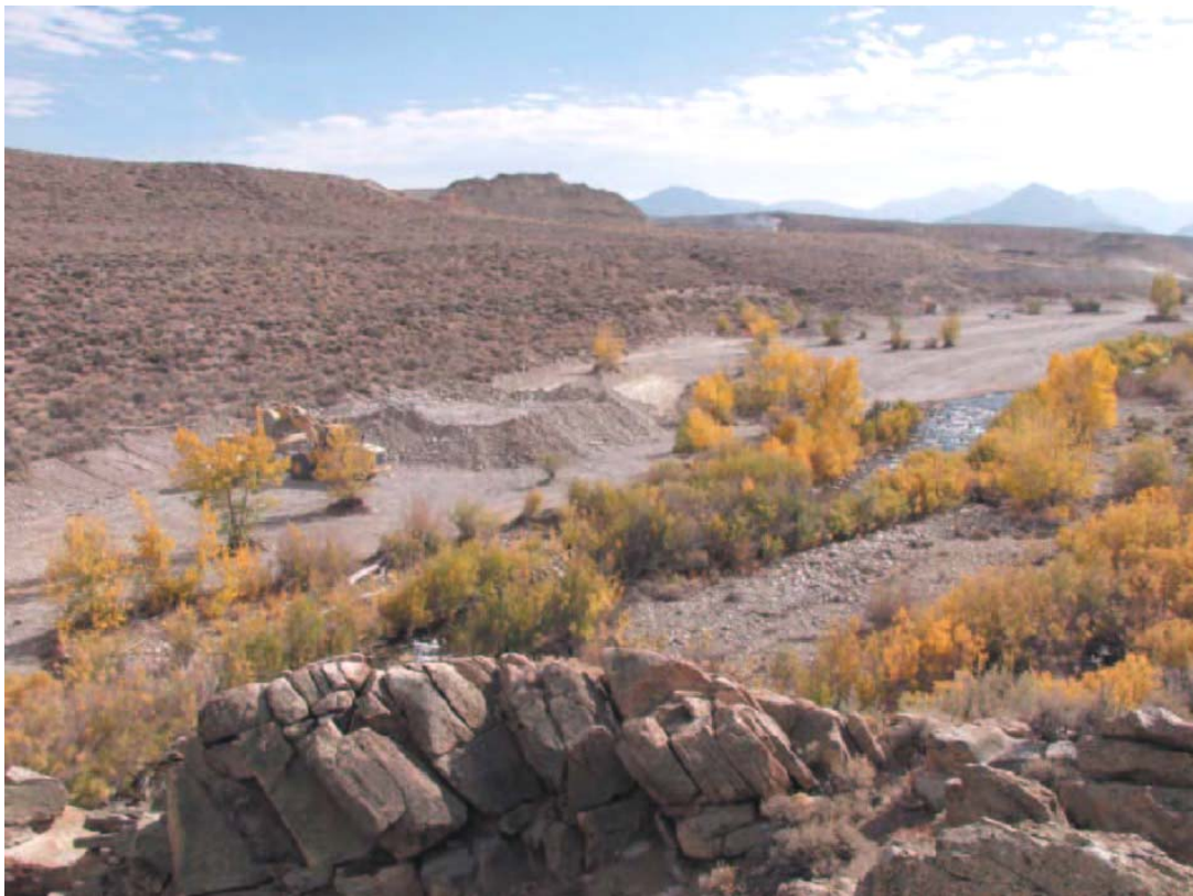
Figure 4: 3D Floodplain Restoration Site: Excavation Completed
