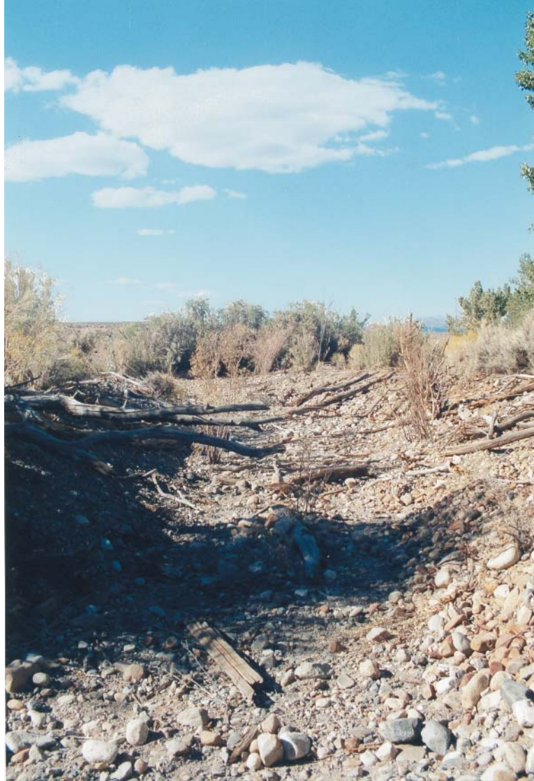
Figure 11. Photograph of the 8-Channel Entrance site looking “downstream” from the entrance to the 8-Channel, prior to construction.
